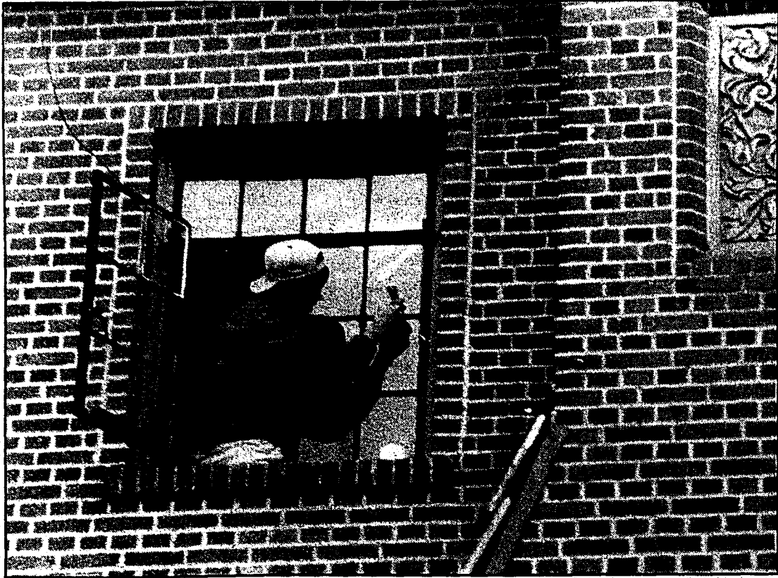
WORKING AWAY. Erik Olsen fixes a window on the second floor at 600 University Ave. (JIM VOLLBRECHT PHOTO)
