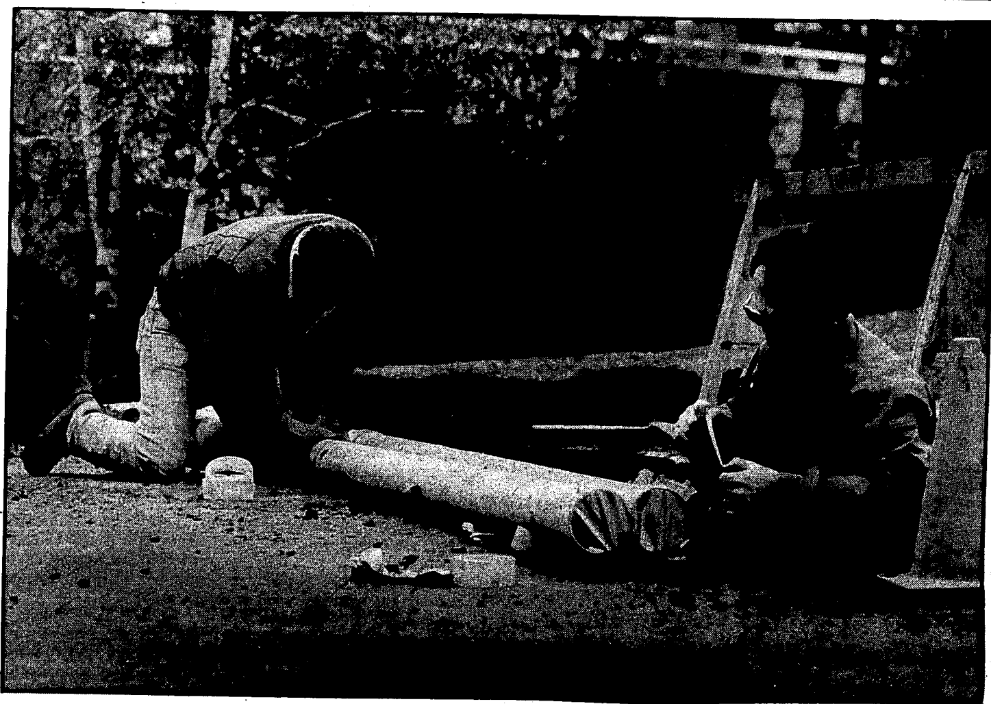
Darrel Hornback (left) and John Veien busy themselves installing communication networks beneath Nez Perce Drive on a cloudy Monday afternoon. (Travis Gadsby PHOTO)
