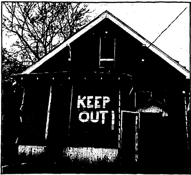
Keep out sign warns people of possible danger. ( Jeff Curtis PHOTO )
