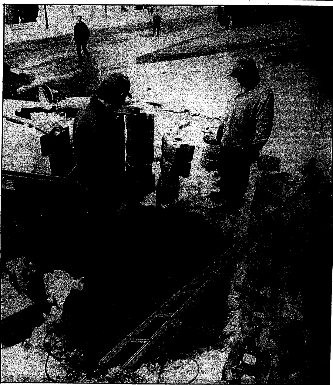
Wayne Anderson and Dave Gray watch and wait while water is pumped out of a manhole where they are doing electrical work. (JEFF CURTIS PHOTO)
