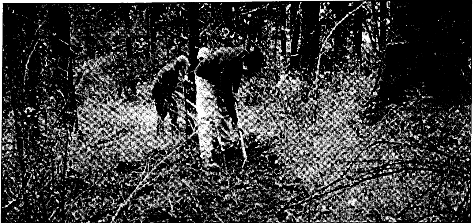
Jeff Johnson (left) and Jon Meir (right) work on moving a trail at Spring Valley Reservoir near Troy, Idaho.
