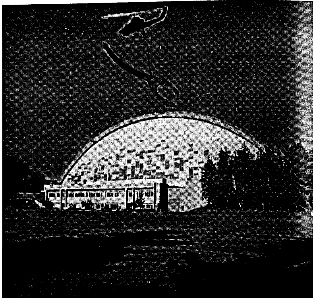
On Saturday, an Apache helicopter flew in a giant can-opener to finish a job the UI should never have started. Fans applauded, fair weather fans wept and concrete tumbled as the roof was finally pried off.
