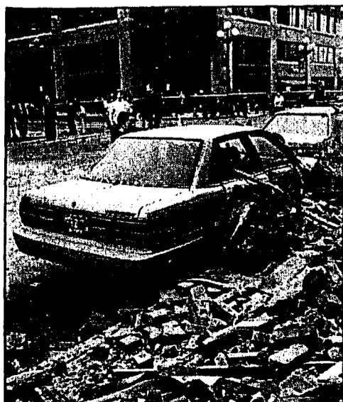
STEVEN MORGAIN / ASSOCIATED PRESS SEATTLE — Kim Yamagiwa examines her car after the wall of a building it was parked next to collapsed during an earthquake in the downtown sector Wednesday.
