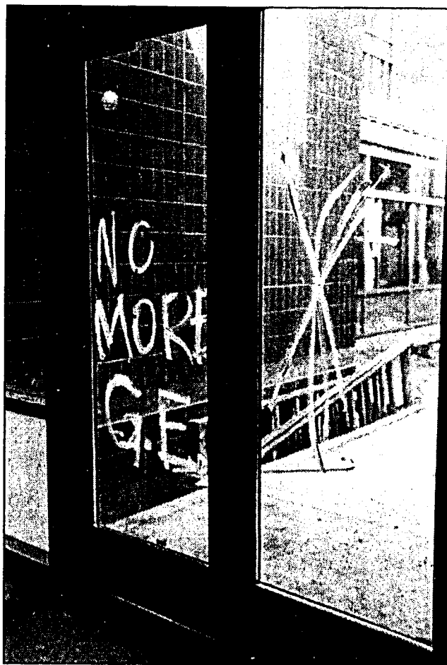
SHAUNA GREENFIELD / ARGONAUT The Ag Biotech Building was vandalized before spring break. Spray paint of anarchy symbols and messages such as "No more G.E." were found throughout the interior of the building, which is still under construction. Police estimate $4,000 in damage.
