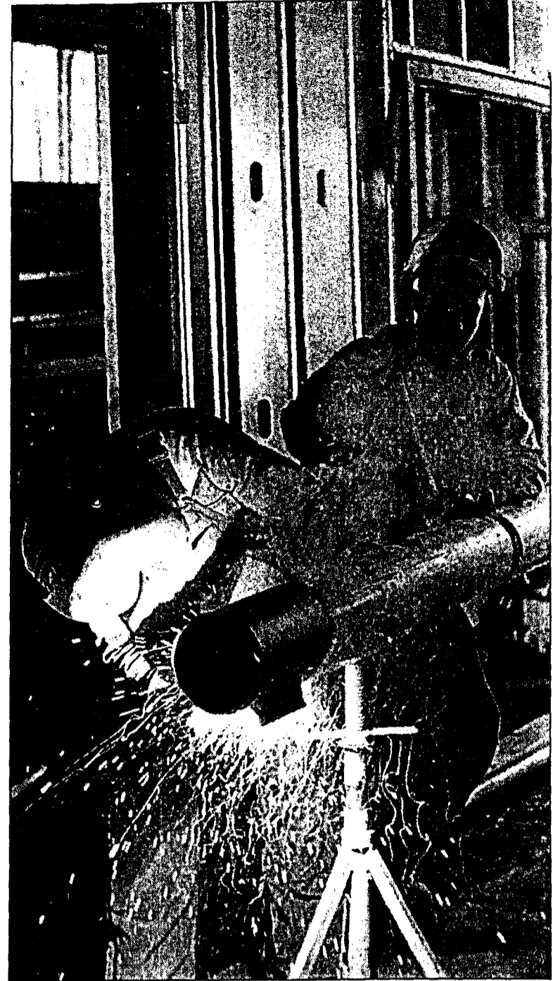
RYAN TOWN / ARGONAUT Dan Huffman, left, and Chris Whitten fit a joint to a pipe that will provide steam to some of the air and water heaters at the University of Idaho Recreation Center. The Rec Center is scheduled to open in February 2002.
