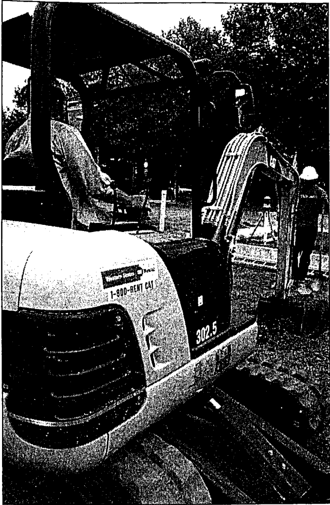
Bill Sigmund, from Motley and Motley construction, is digging footings for the new resident halls Wednesday.
