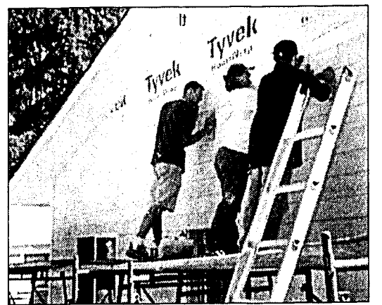
JESSICA LIPSCHULTZ / ARGONAUT Nathan Beach, Katie Wittman-Conklin and Mason Fuller paint a Habitat for Humanity home in Genesee. Wittman-Conklin is the current AmeriCorps *VISTA volunteer for community service programs at UI.
