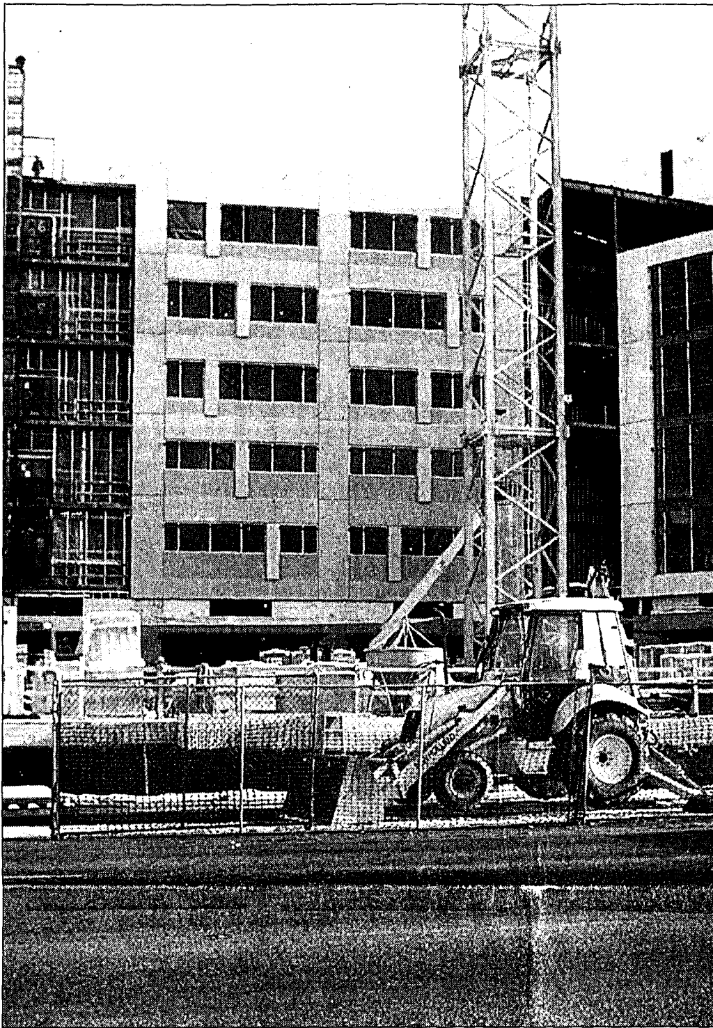
JUDY LOSTROM / SPECIAL TO THE ARGONAUT Work progresses at the Idaho Water Center in Boise.
