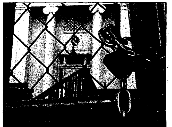
The Sigma Nu fraternity house, which has been empty since Christmas break, is currently being remodeled.
