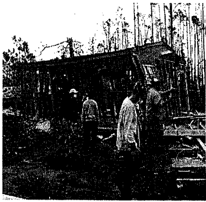
U of I students knock over a building demolished by Hurricane Katrina.
