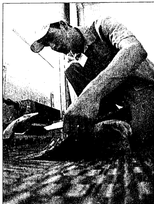
Kentaro Murali/Argonaut Temporary custodial staff member and senior Joel Baillinger installs carpet squares in a new concept room Friday in the Gooding Wing of Wallace Residence Center.
