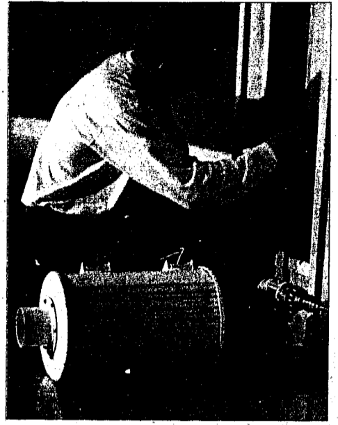
Jake Barber/Argonaut Mark McCully from Q C Electric installs a light fixture in the newly renovated Student Union Building Ballroom Thursday.
