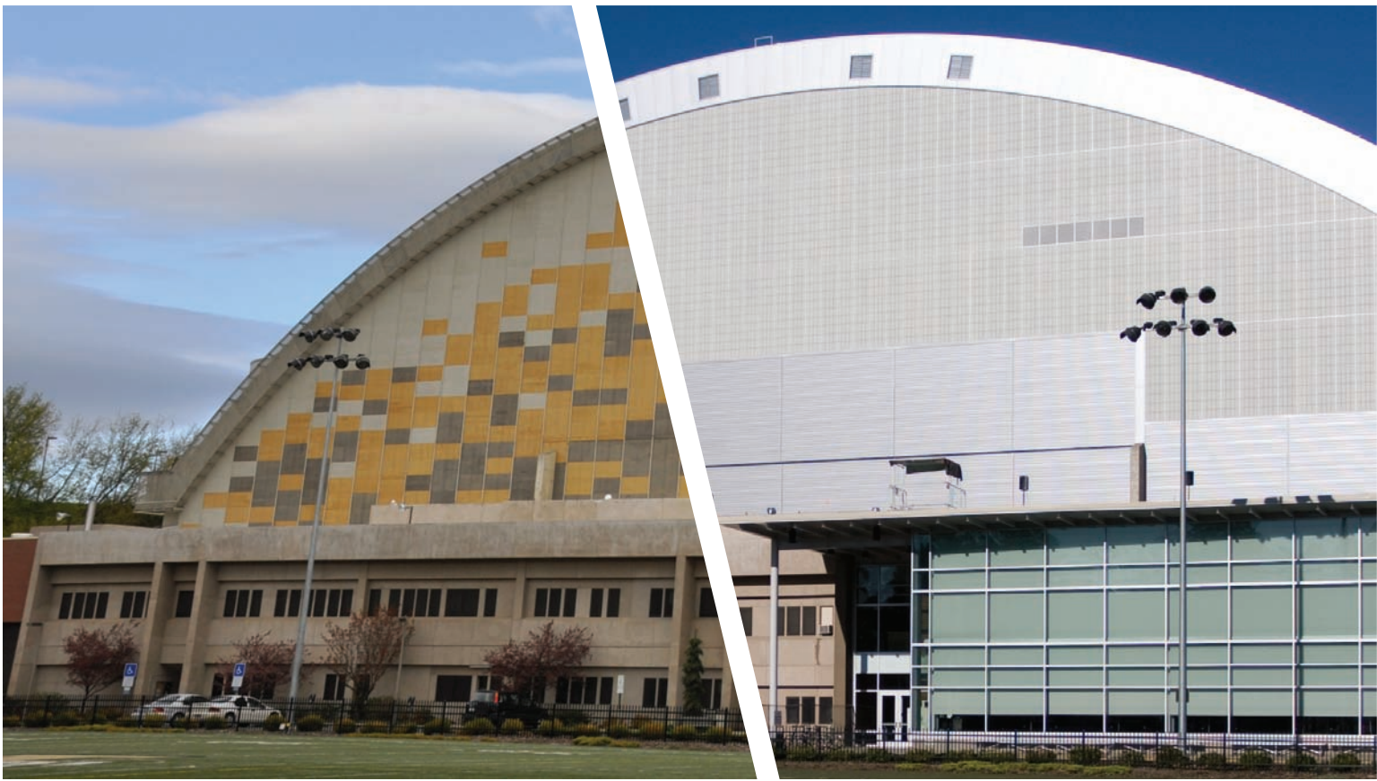
Left photo taken spring 2010 before exterior construction, right photo taken fall 2011 following completion of renovations. Complete construction took a total of three years and cost approximately $28 million.
