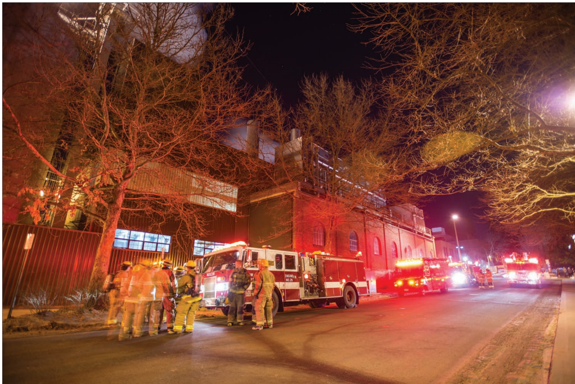
The Moscow Volunteer Fire Department responds to a call concerning the University of Idaho Steam Plant at 8:50 p.m. Monday on Line Street. "A passerby saw steam coming out of a window of the steam plant. They thought it was smoke and reported a fire," said Lt. Dave Lehmitz of the Moscow Police Department. No fire was found at the scene. Philip Vukelich | Argonaut
