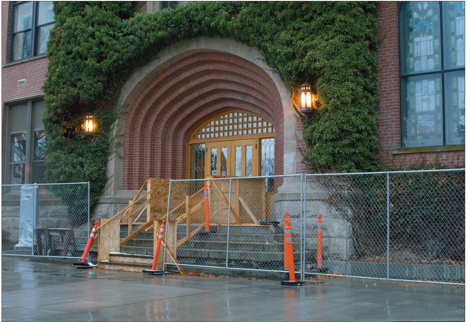
The north entrance of the Administration Building under construction.
