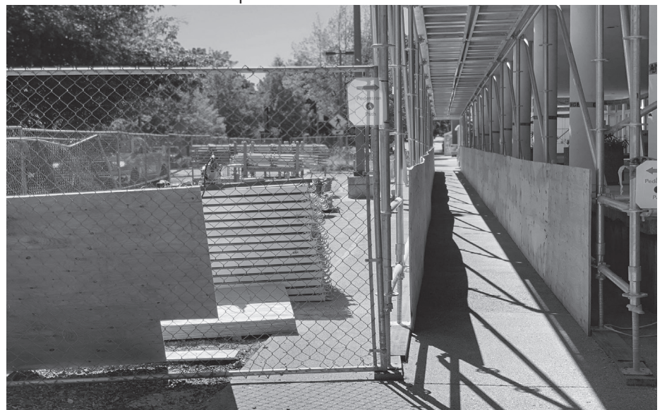
Construction at the Bruce Pitman Center.
