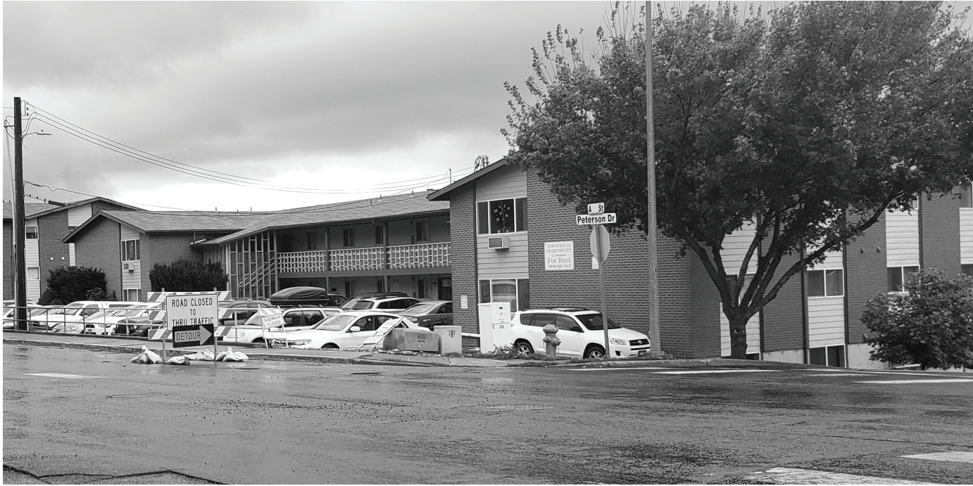
Construction on A Street near intersection with Peterson Drive Oct. 21.
