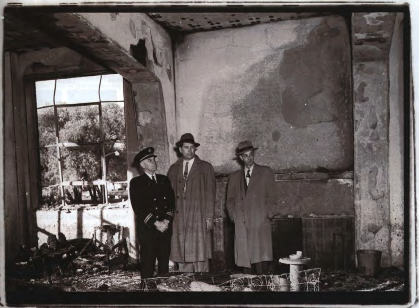
Gault Hall fire [1956]. Lounge on second floor where fire broke out. 1-95-2. University of Idaho Library
