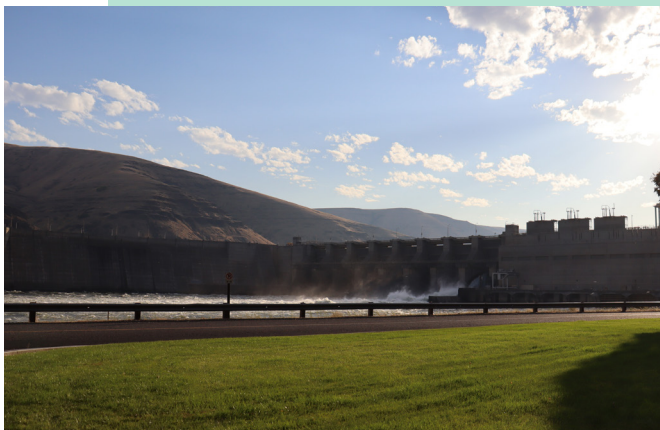
CONSTRUCTION OF THE LOWER GRANITE LOCK AND DAM FINISHED IN 1975, IT WAS THE FOURTH DAM PUT ON THE LOWER SNAKE RIVER.
