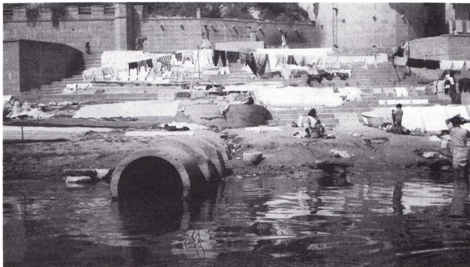
Sewage pipe in the Ganges River
