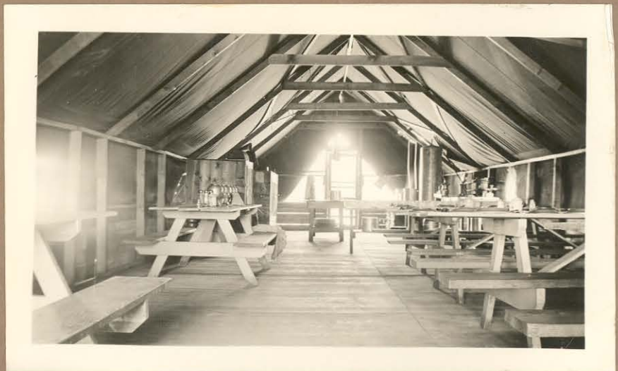
Interior of Mess Hall at Box T Spike Camp
