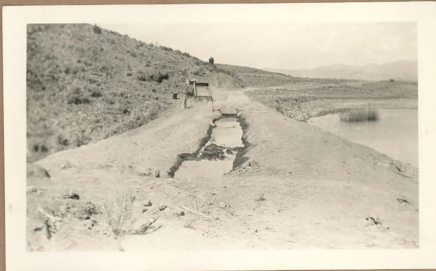
Showing Puddle-Core on Spencer Dam.
