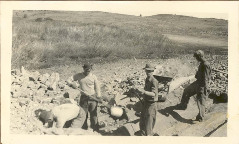
Rock excavation by hand tools and wheelbarrow.
