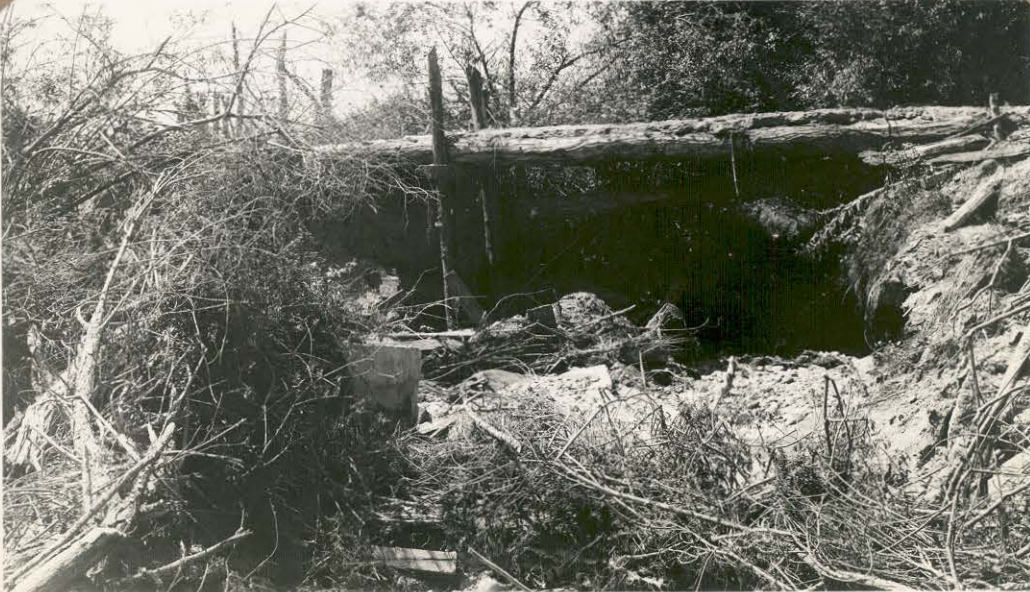
The result of water not controlled.
