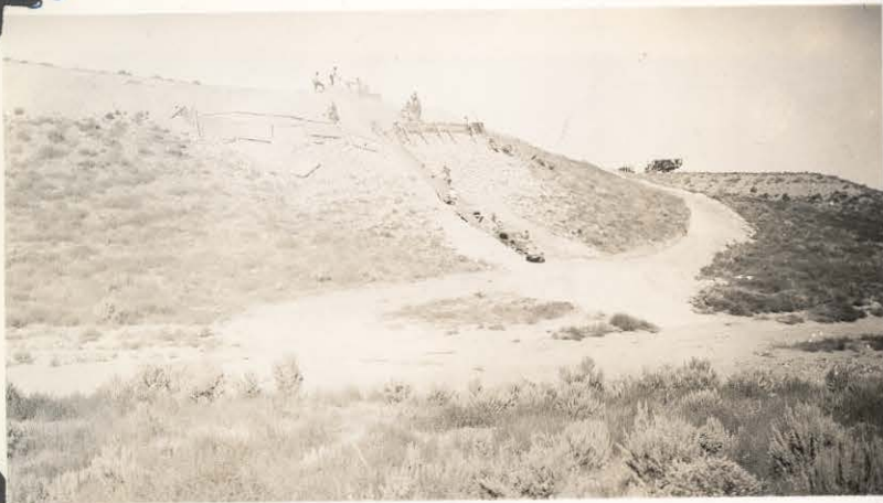
Three ways of loading gravel; No 1 Teams, ramp, and truck. No 2. Shoveling into chute. No3. Bulldozer replenishing gravel pit.
