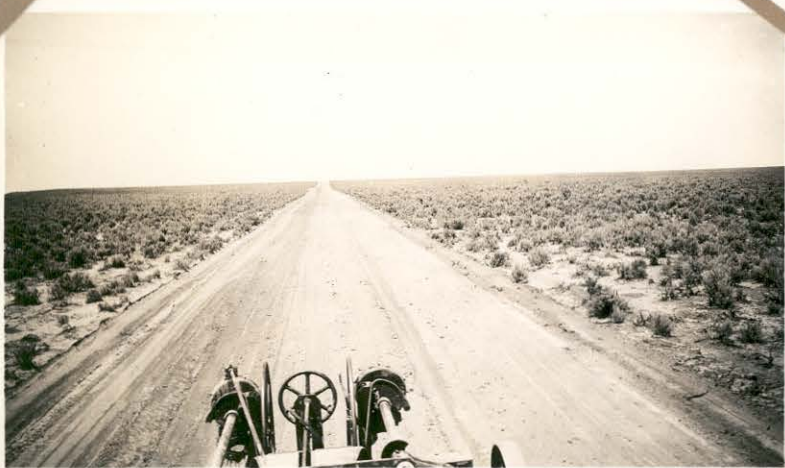
PROJECT NO. 1--HOT SPRINGS WINTER CAMP ROAD, 21 MILES.
