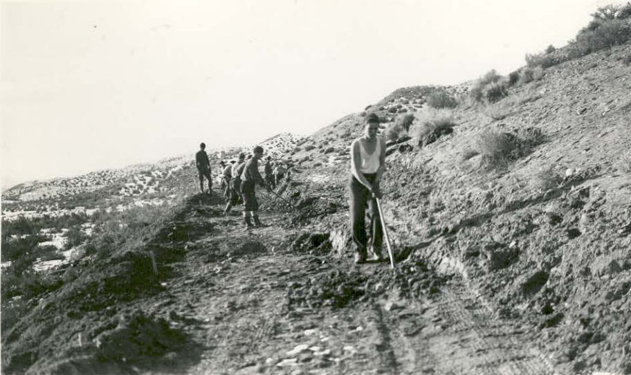
Showing Excavation with hand tools
