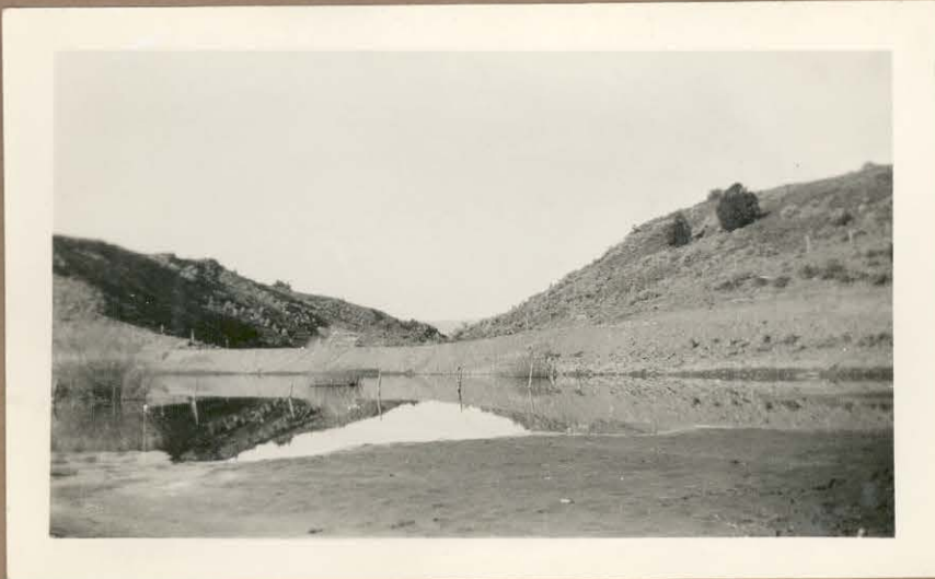
Showing old reservoir before drainage. Taken shortly after work was commenced on Dam
