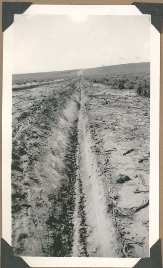
After all sagebrush was removed, the caterpillar, bulldozer, and grader went into operation, leaving a surface that is high and dry for year around travel.
