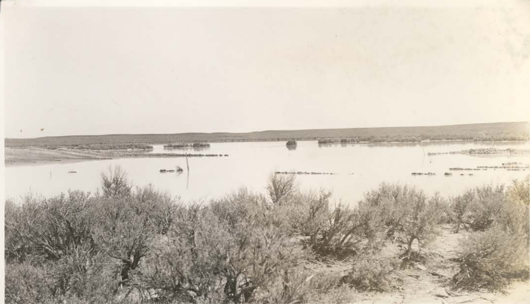
No. 2. Dry Lake No. 1. Now under construction. Located in Sunnyside desert.
