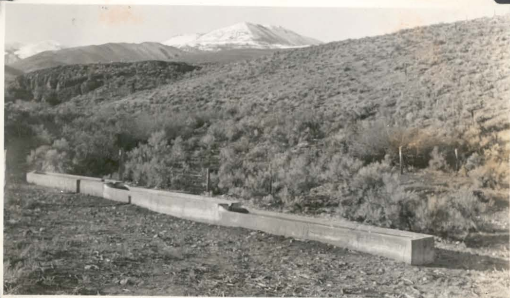
Side view of the Bates Creek cement water troughs For details see reverse side
