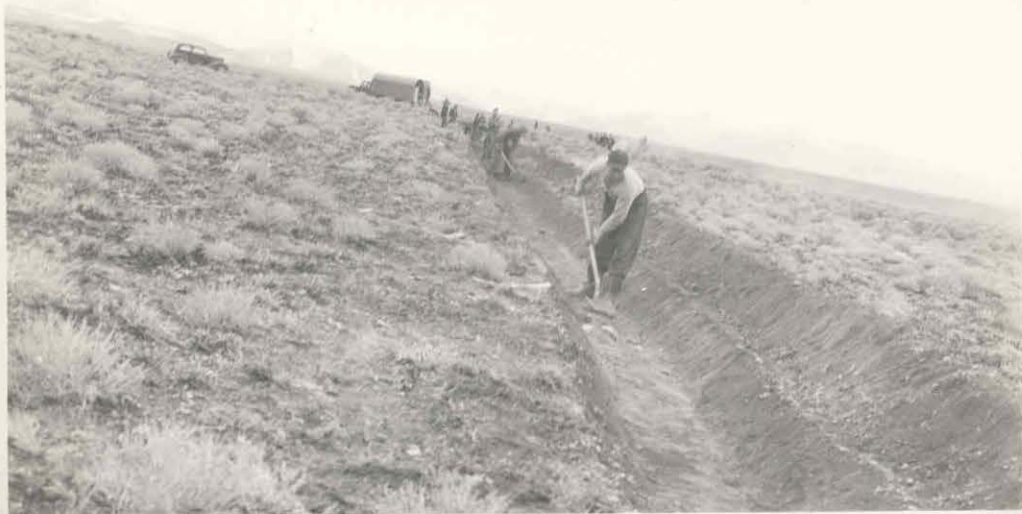
No. 1 Digging feed ditches, which will supply reservoirs with summer water.
