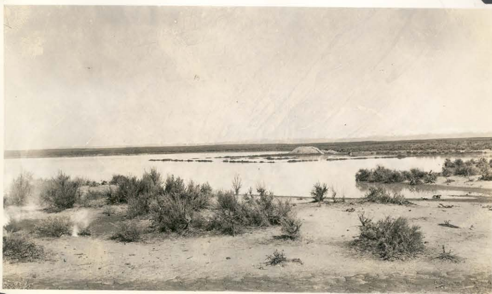
No. 3. Dry Lake No. 1. Now under construction. Located in Sunnyside desert.
