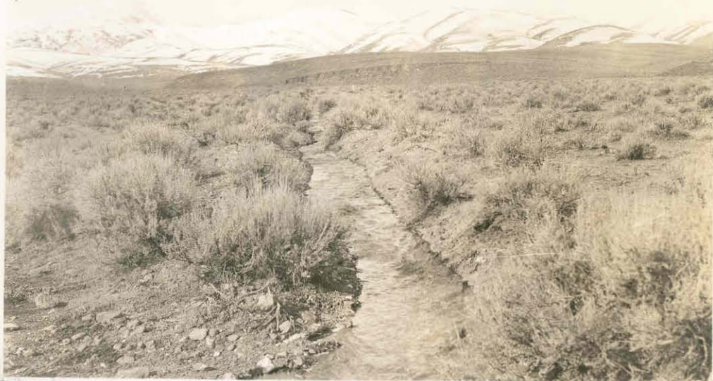
No. 2. A completed ditch, which has filled reservoirs No. 5-6 and one below.
