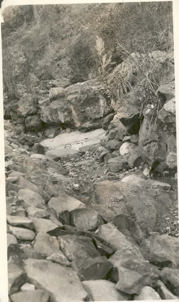
Bates Creek Spring Re-enforced- Concrete Top & sides with man hole
