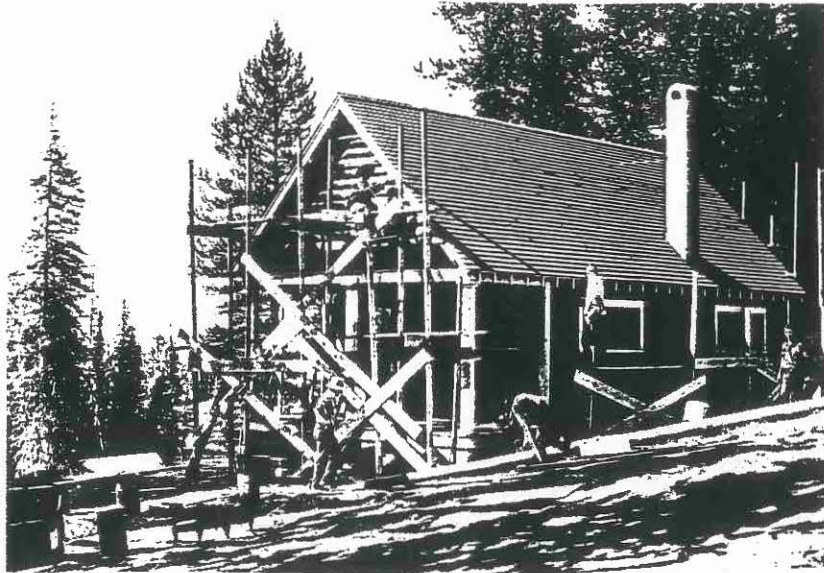
Fig. 1 Trinity Lakes Guard Station dwelling under construction, 1933.
