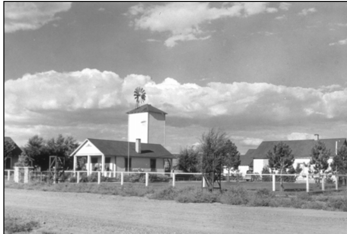
Plan 51 Office, Plan 21 Garage and other standard buildings, Paradise Valley Ranger Station, Humboldt-Toiyabe National Forest
