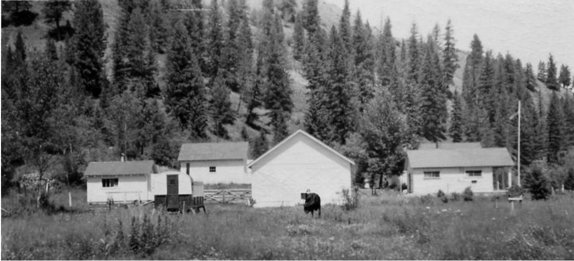
Copper Creek Ranger Station (Cobalt Summer Administrative Site), 1948. Photo courtesy of Philip Gutzman. Mr. Gutzman lived on site while his father was ranger. He identified the pile of rocks on the left as the cellar and the adjacent building as the blacksmith shop. The summer smokechaser stayed in the "pie wagon" in the left foreground. On the right, two small posts with a rail held the rain gauge. The cow belonged to the Gutzmans.
