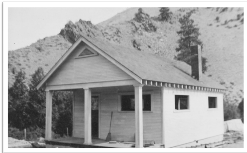
R4 Plan 7 under construction at Williams Creek Guard Station
