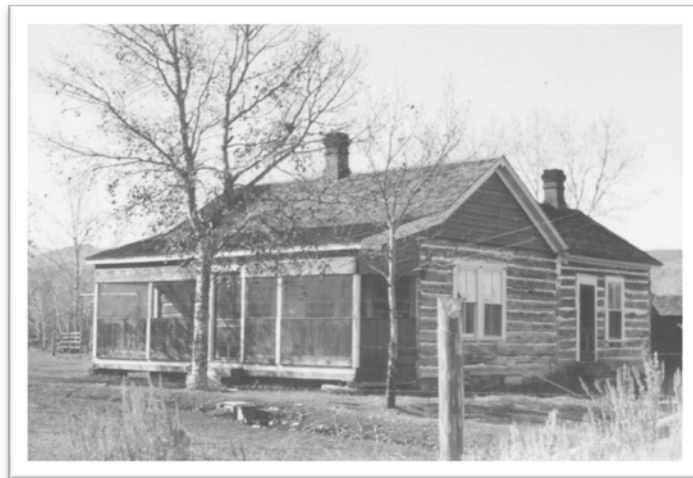
Lemhi Ranger Station Office/Dwelling
