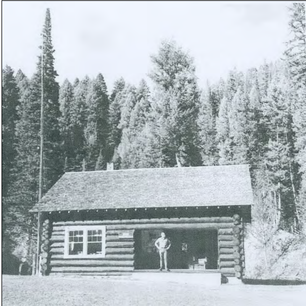
1963 photo of the east (front) wall of the combination building. Note the recessed loading dock, which should have been at the rear of the building. (HF BNF)
