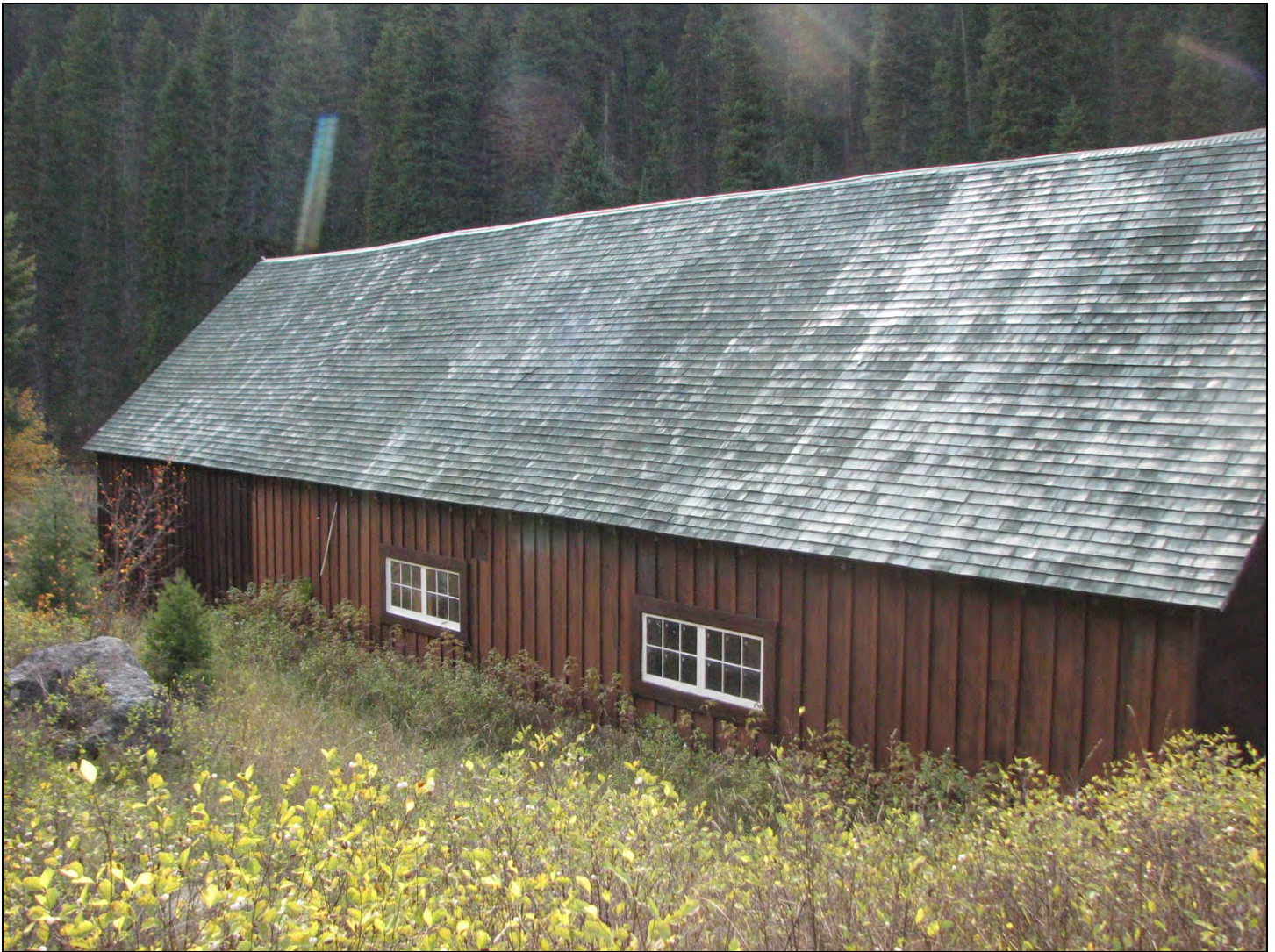
Photo 0019 Looking south-southwest at the east (rear) wall of the garage / shop.
