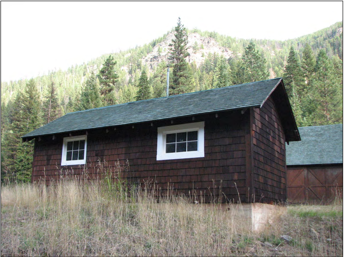
Photo 0021 Looking east-northeast to the west (side) and south (rear) wall of the flammable materials shed.
