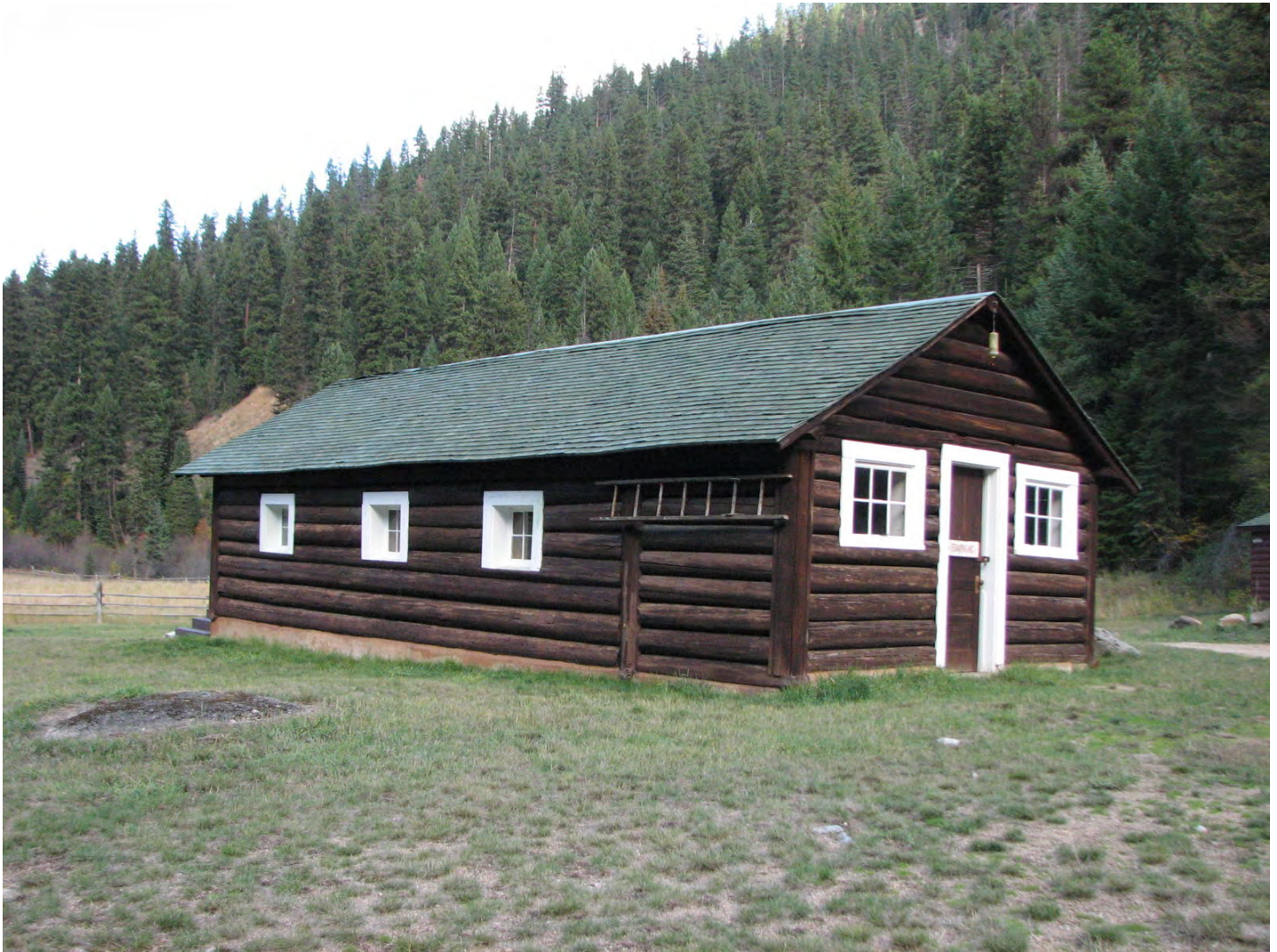
Photo 0017 Looking northeast to the west (side) and south (rear) walls of the fire cache.
