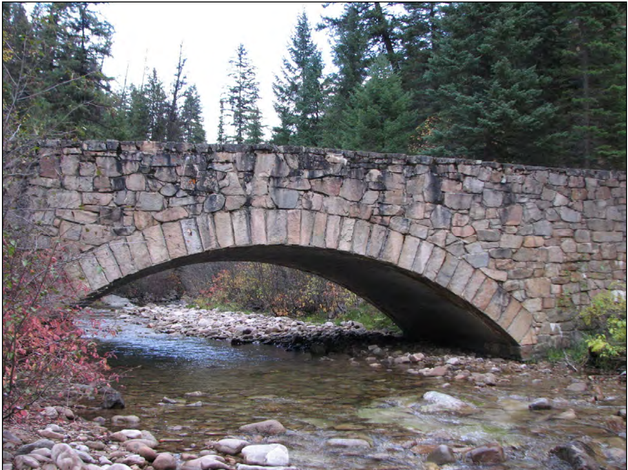
Photo 0006 Looking northeast at the west face of the Deep Creek Bridge.
