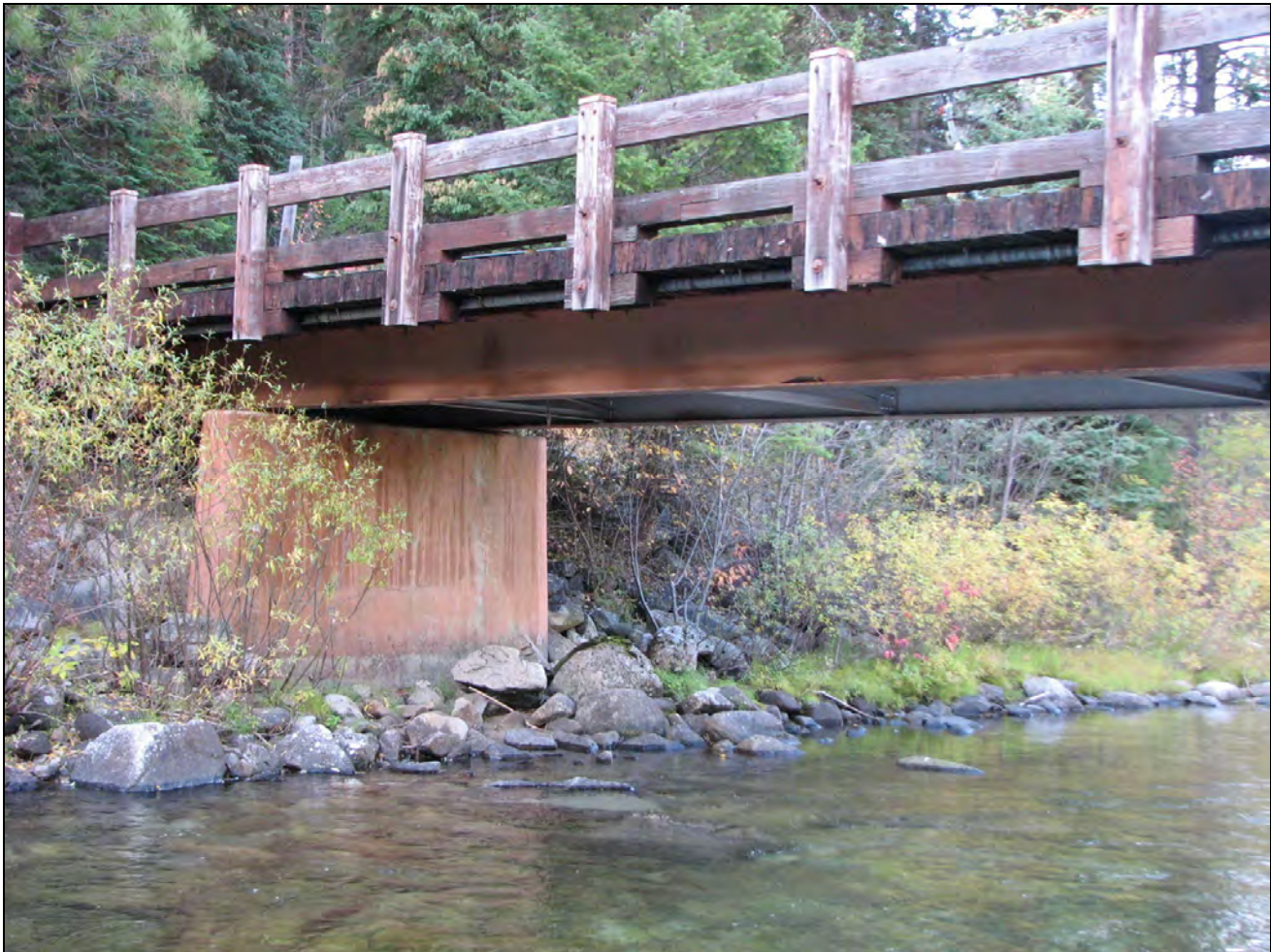
Photo 0008 Looking north-northwest to the I-beam bridge.
