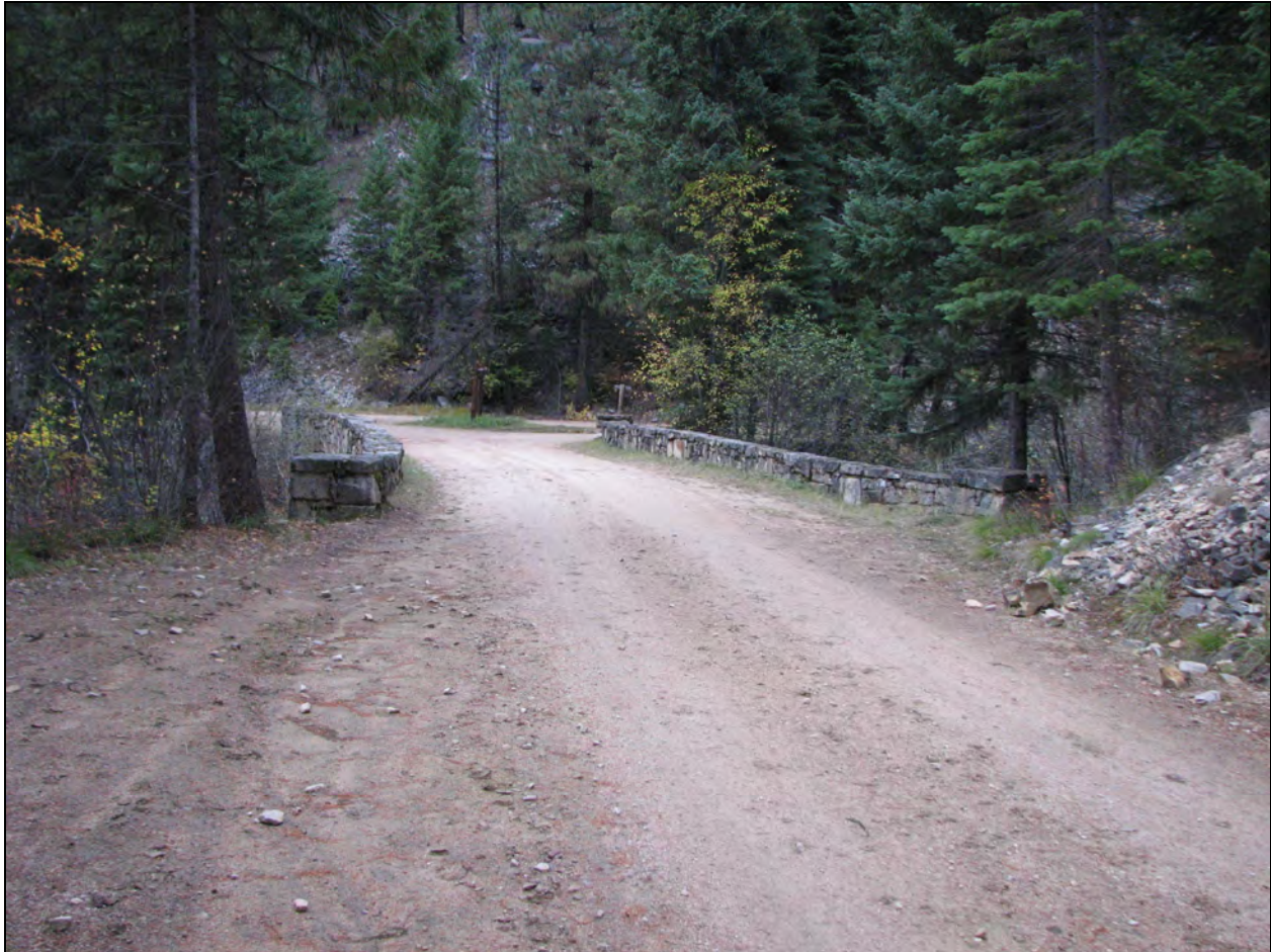
Photo 0005 Looking northeast across the running surface of the Deep Creek Bridge.
