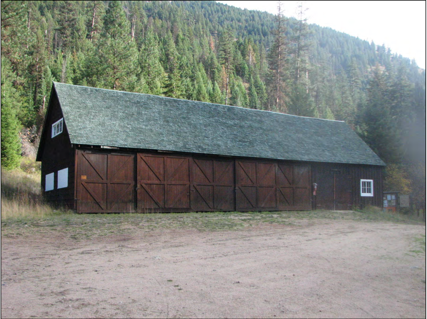
Photo 0018 Looking east-southeast to the north (side) and west (front) walls of the garage / shop.
