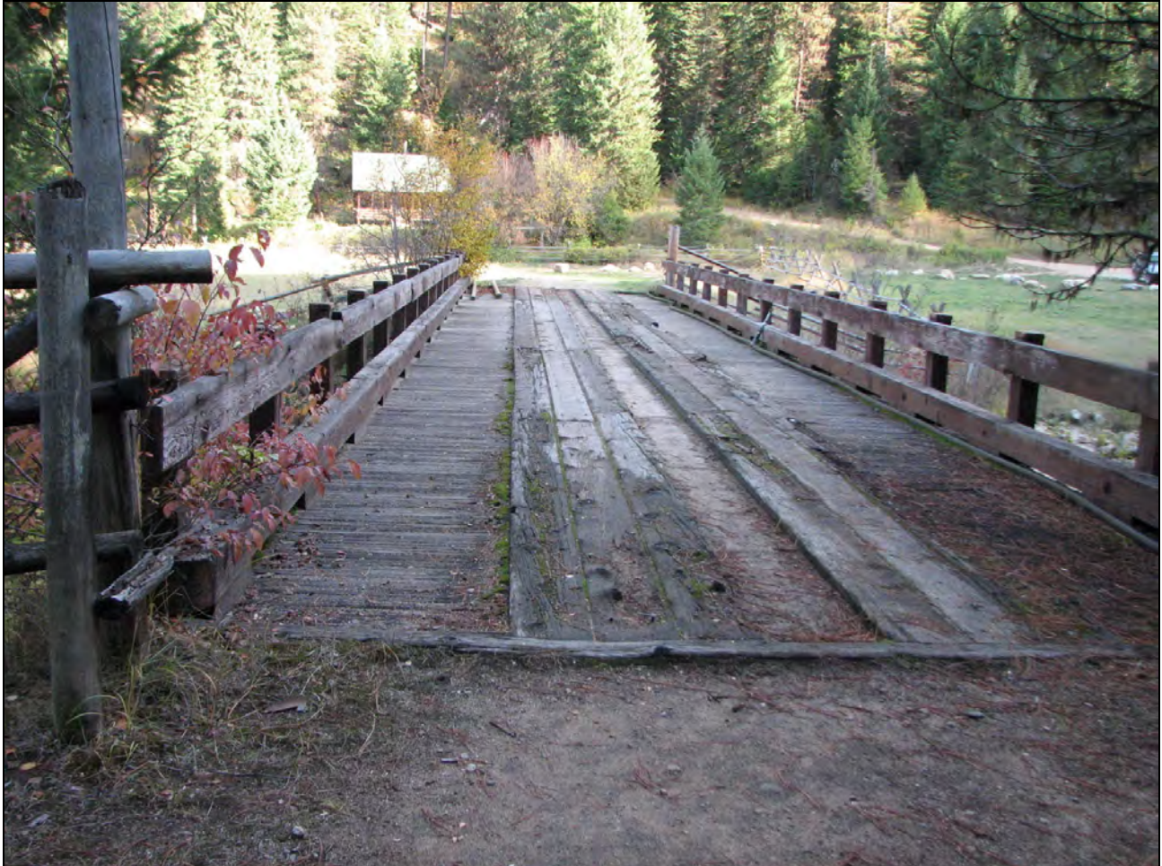
Photo 0007 Looking east across the I-beam bridge.
