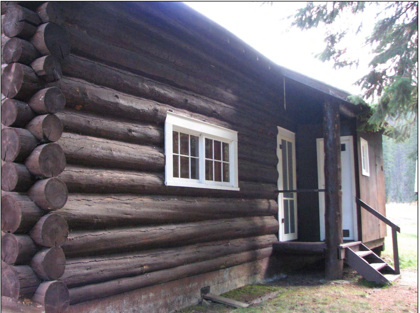
Photo 0013 Looking south-southeast to the west (rear) wall of the combination building.
