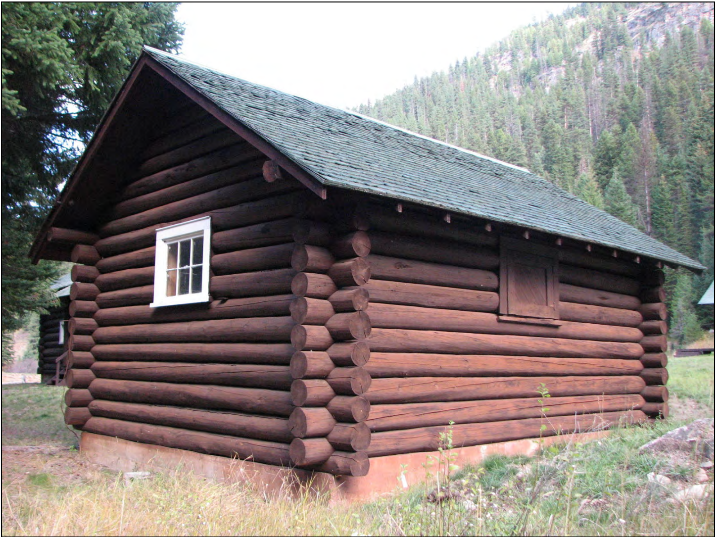
Photo 0015 Looking northeast to the west (side) and south (rear) walls of the wood shed.
