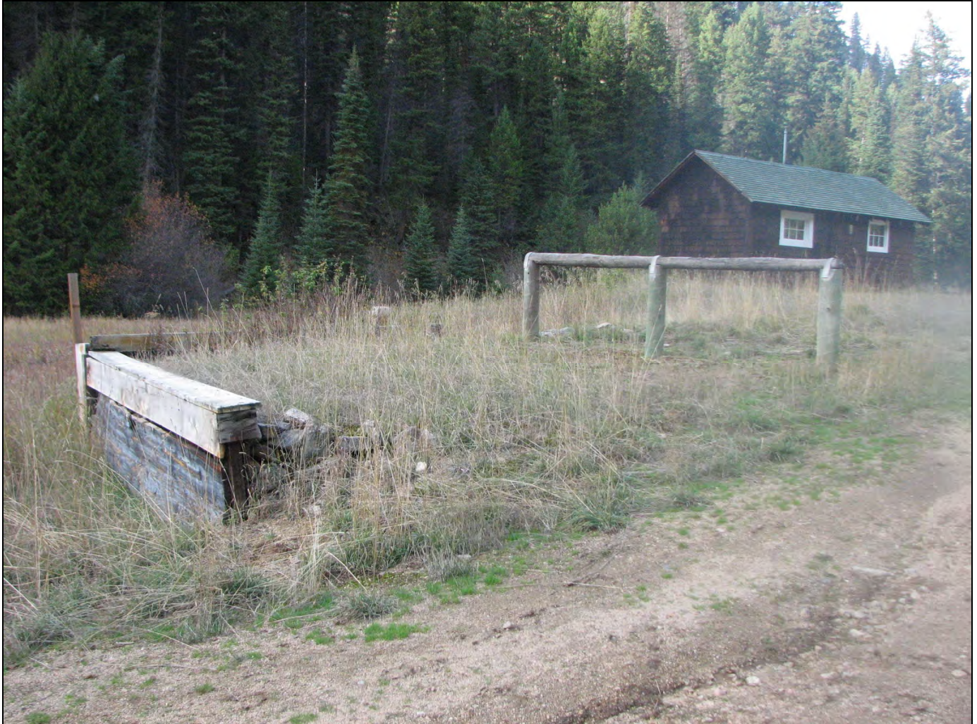
Photo 0026 Looking northwest to the stock loading platform and hitching rail near the garage / shop
