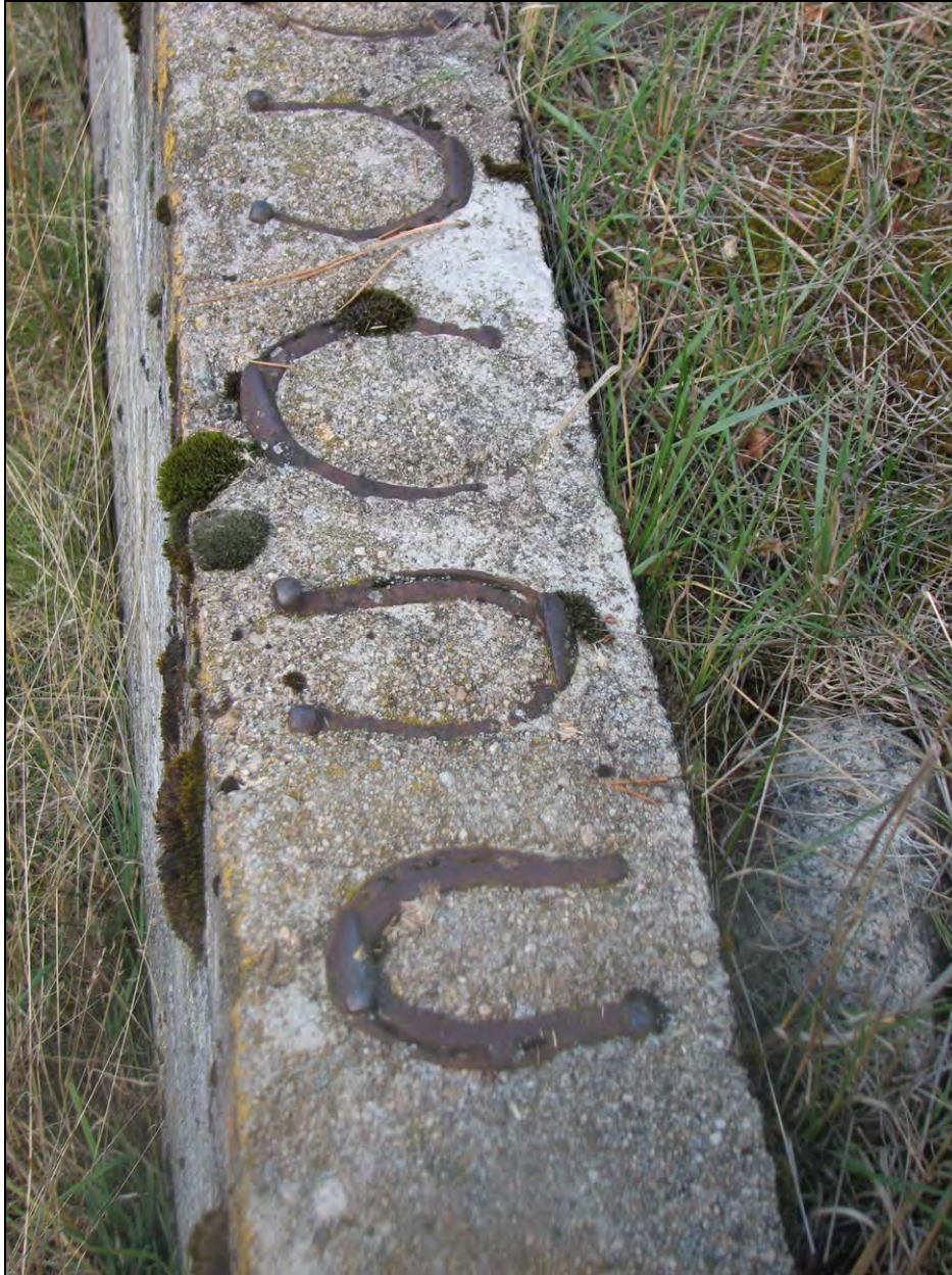
Photo 0027 Detail photo of the mule and horse shoes embedded in the stock loading ramp adjacent to the Barn.
