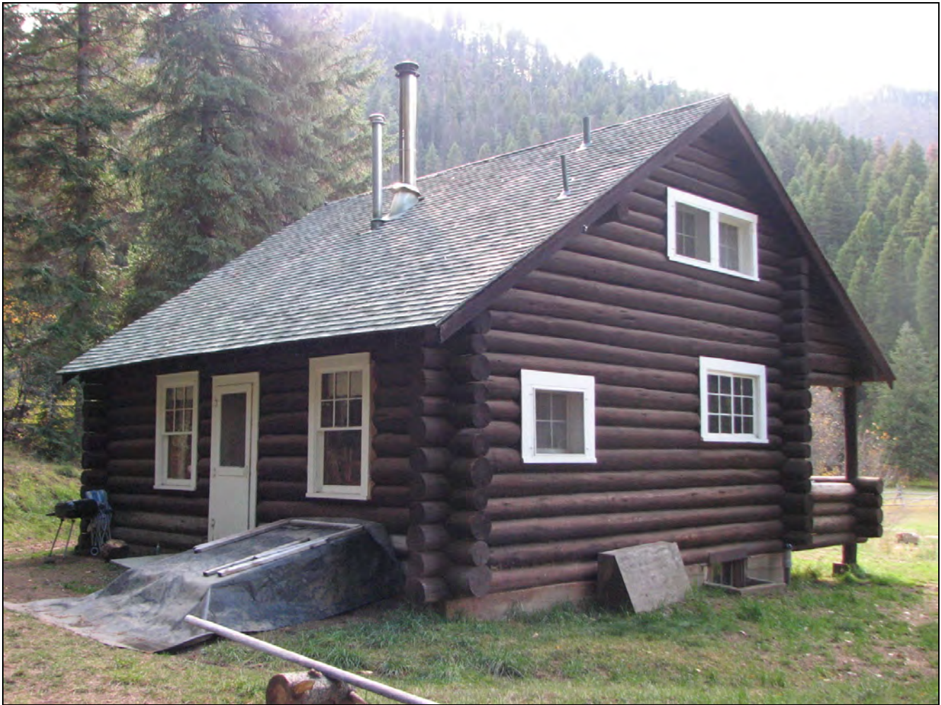
Photo 0010 Looking southwest to the east (rear) and north (side) walls of the ranger's dwelling
