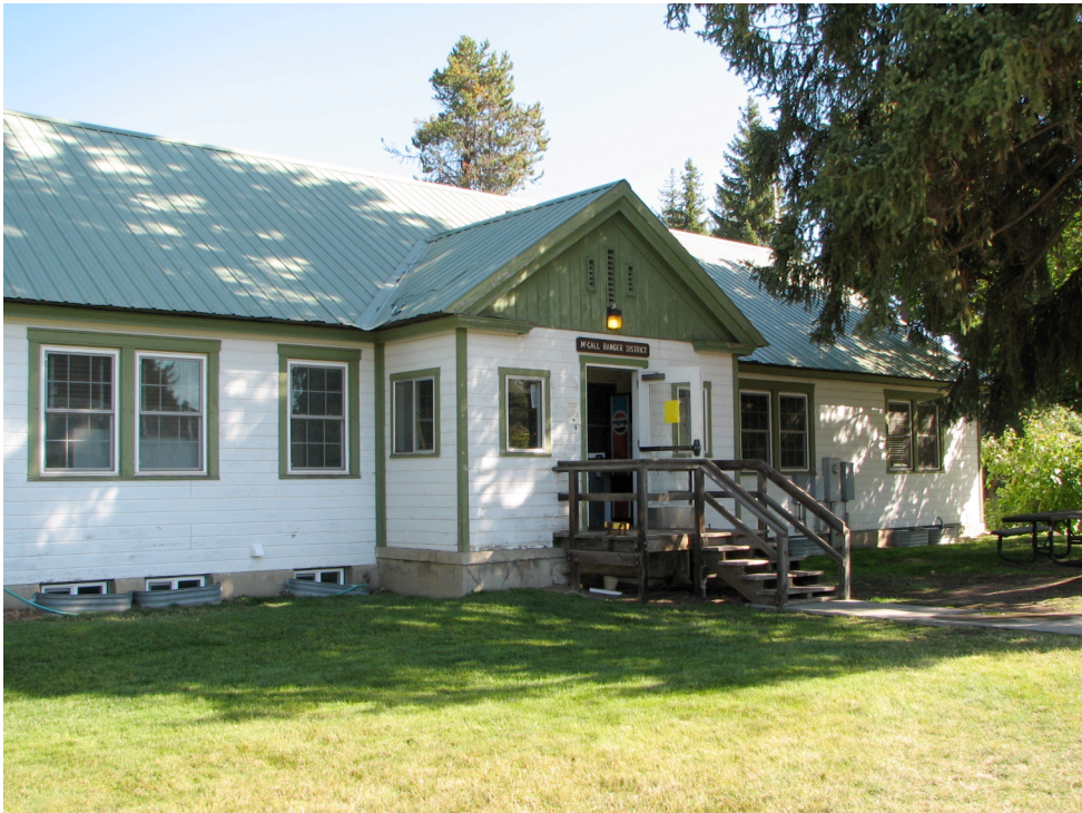
Figures 11a and 11b. The north and west sides (top) and the south side (bottom) of Building I, the McCall District Office (#1201), McCall District Administrative Site, 2008.
