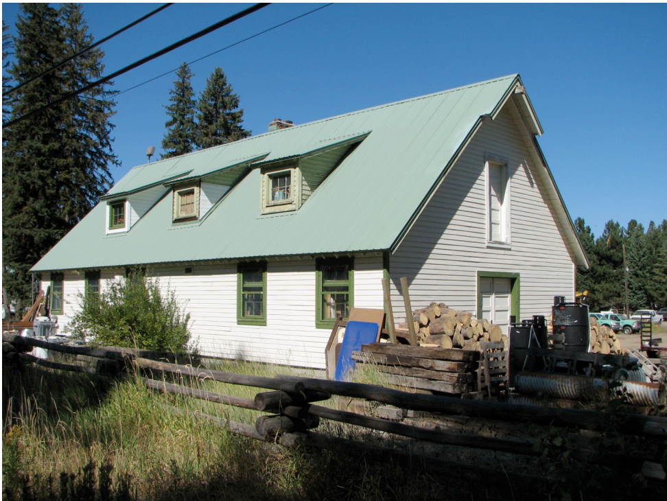
Figures 5a and 5b. The north and west sides (top) and the south and east sides (bottom) of Building B, the McCall District Warehouse (#1503), McCall District Administrative Site, 2008.
