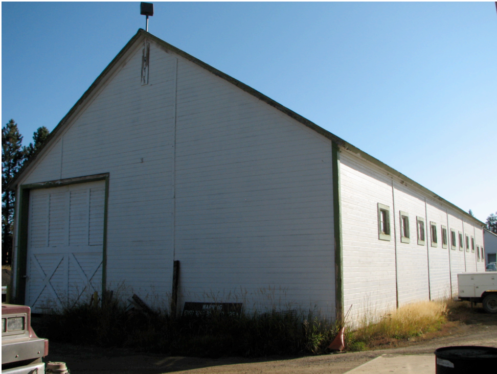
Figures 4a and 4b. The east and north sides (top) and the west and south sides (bottom) of Building A, the Hay Barn (#1320), McCall District Administrative Site, 2008.
