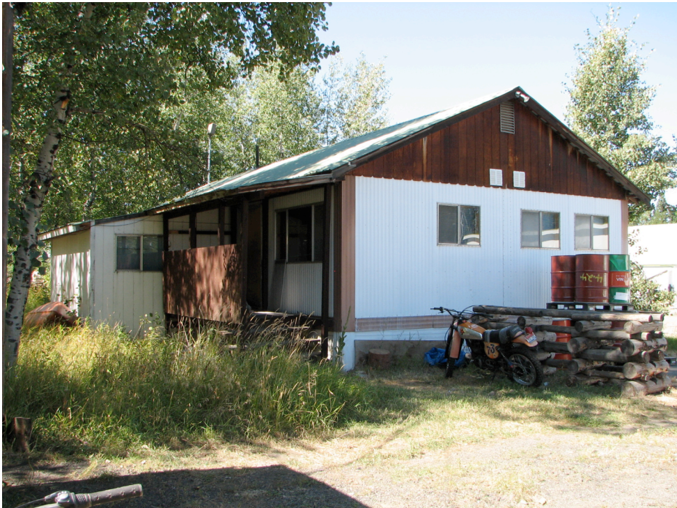
Figures 13a and 13b. The north and west sides (top) and the south and east sides (bottom) of Building K, the Land Line Surveyor's Building (#1212), McCall District Administrative Site, 2008.
