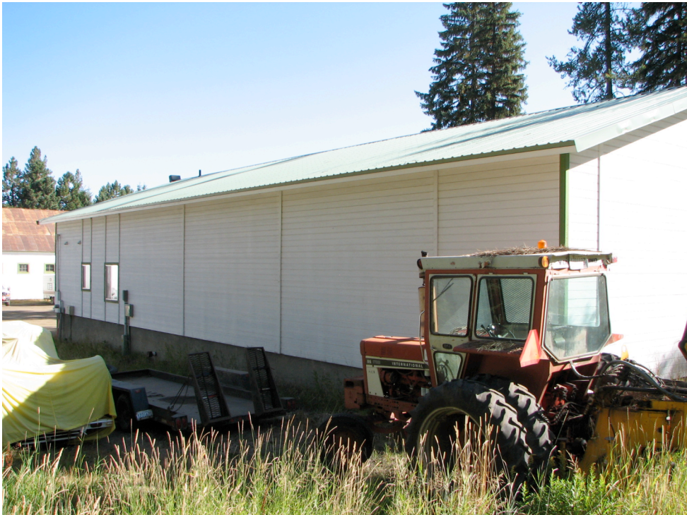
Figures 17a and 17b. The east and north sides (top) and the west side (bottom) of Building 2, the Tree Cooler Building (#1392), McCall District Administrative Site, 2008.
