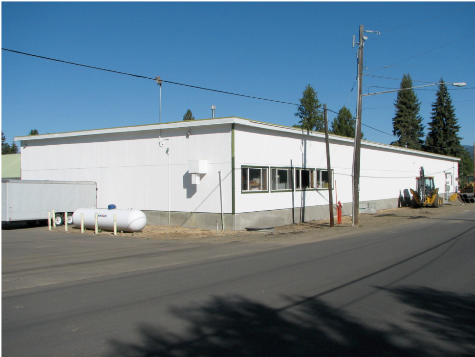
Figures 12a and 12b. The north and west sides (top) and the south and east sides (bottom) of Building J, the Fire Warehouse (#1304), McCall District Administrative Site, 2008.
