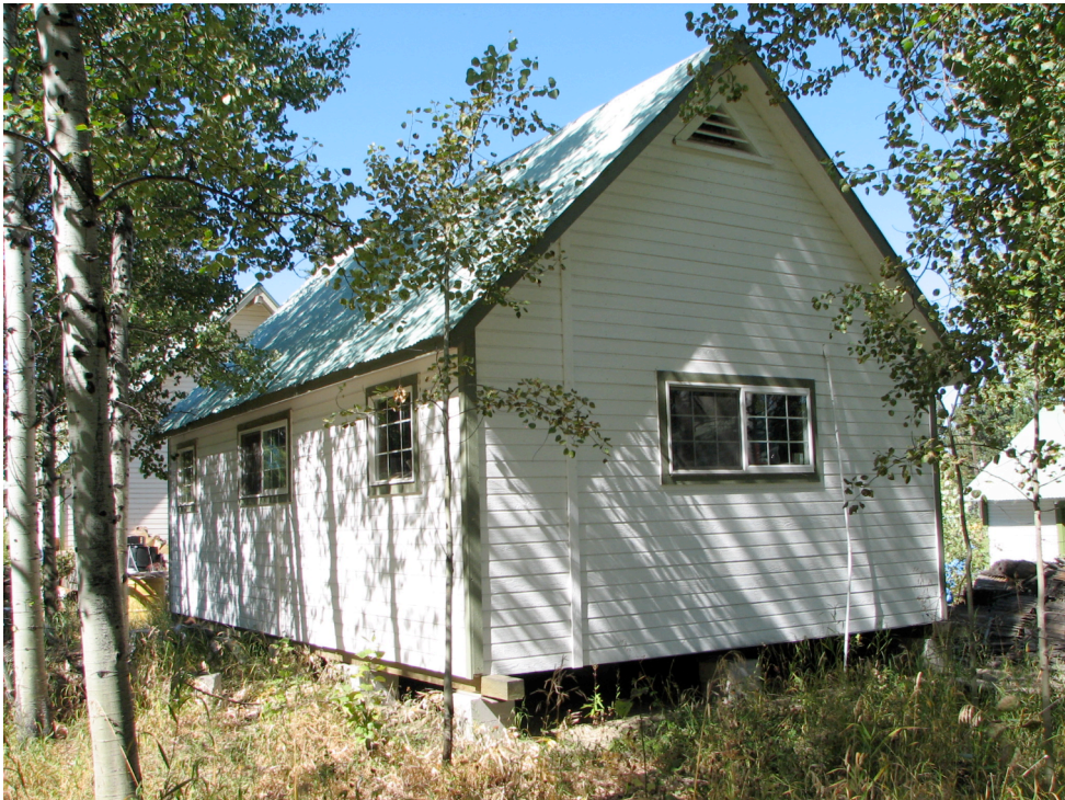
Figures 8a and 8b. The north and west sides (top) and the south and east sides (bottom) of Building E, the Krassel Warehouse (#1205), McCall District Administrative Site, 2008.
