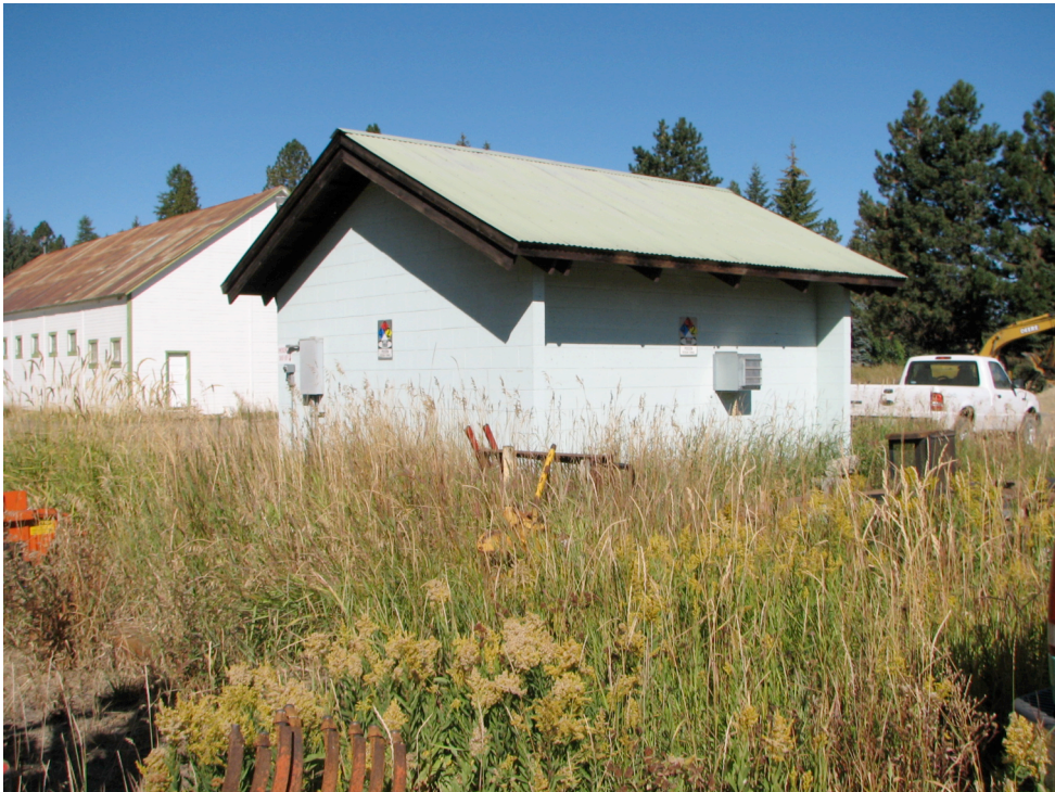
Figures 15a and 15b. The north and west sides (top) and the south and east sides (bottom) of Building M, the Pesticide Storage Building (#1383), McCall District Administrative Site, 2008.
