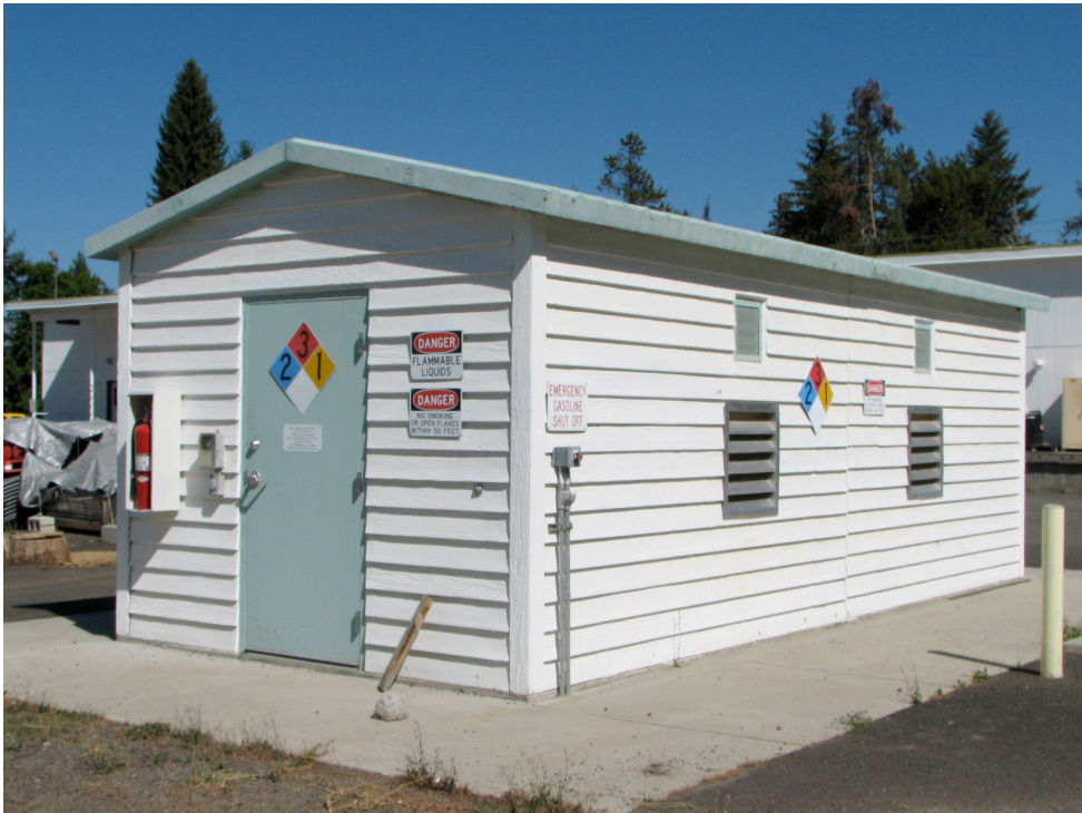
Figures 21a and 21b. The east and north sides (top) and the west and south sides (bottom) of Building 7, the Petrochemical Storage Building (#1431), McCall District Administrative Site, 2008.
