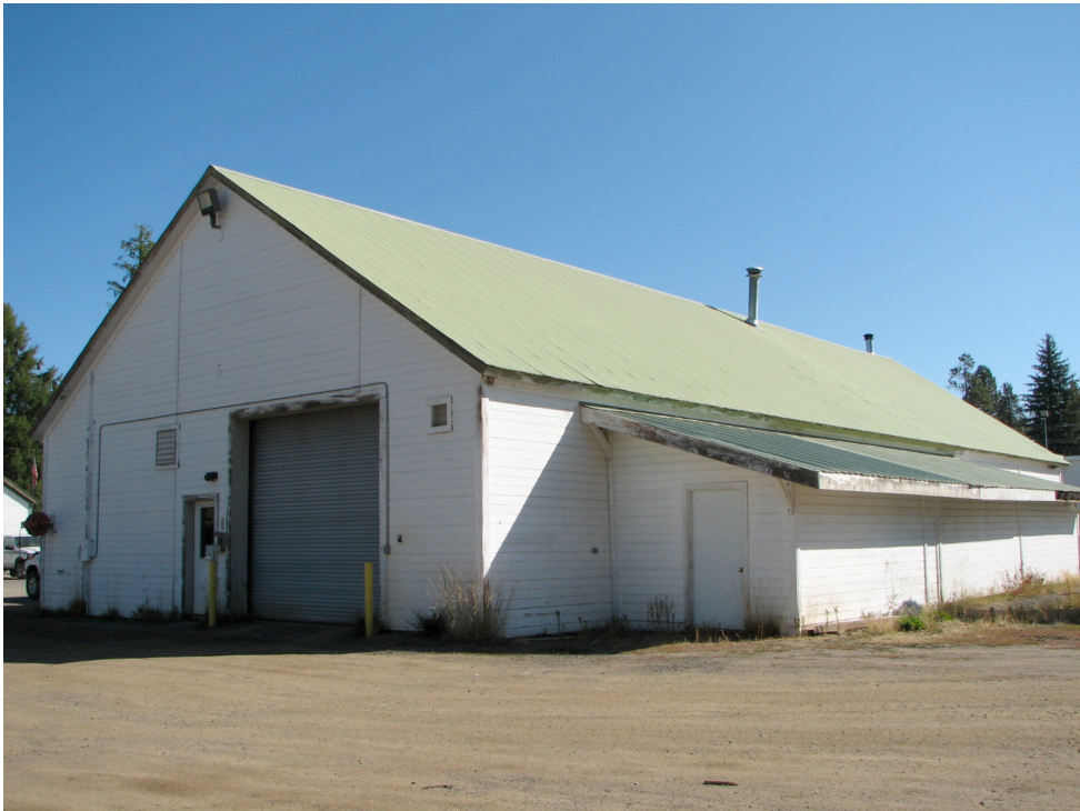
Figures 6a and 6b. The east and north sides (top) and the west and south sides (bottom) of Building C, the Carpenter Shop (#1336), McCall District Administrative Site, 2008.
