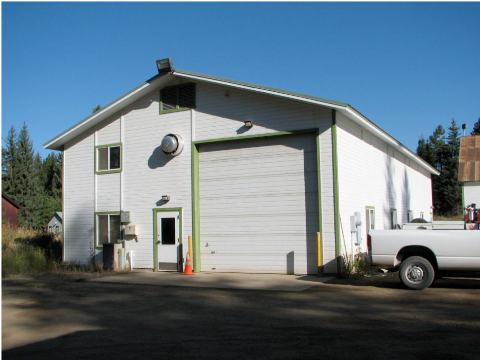
Figures 16a and 16b. The north and west sides (top) and the south and east sides (bottom) of Building 1, the C and M Heavy Machinery Maintenance Shop (#1509), McCall District Administrative Site, 2008.
