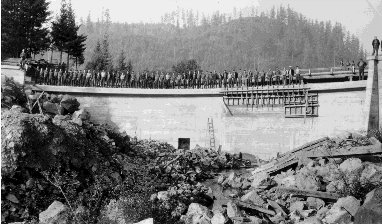
Figure 22. CCC-built dam, Trout Creek, Columbia National Forest. Courtesy of Gifford Pinchot National Forest Heritage Program.
