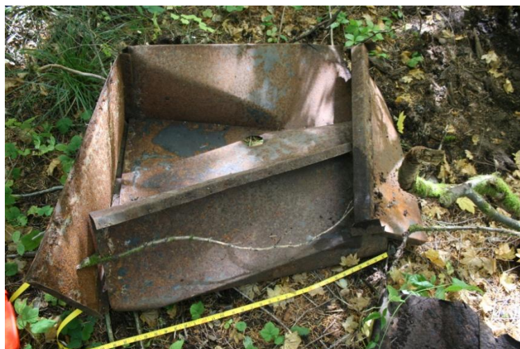
Figure 50. Remains of sink from washroom with wood frame gone. Photograph taken by Matthew Mawhirter October, 2010.
