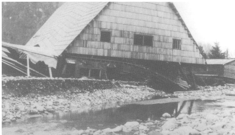
Figure 13. First A-frame recreation hall built at Camp Lower Cispus. Destroyed in a flood in 1933. Courtesy of Gifford Pinchot National Forest Heritage Program.
