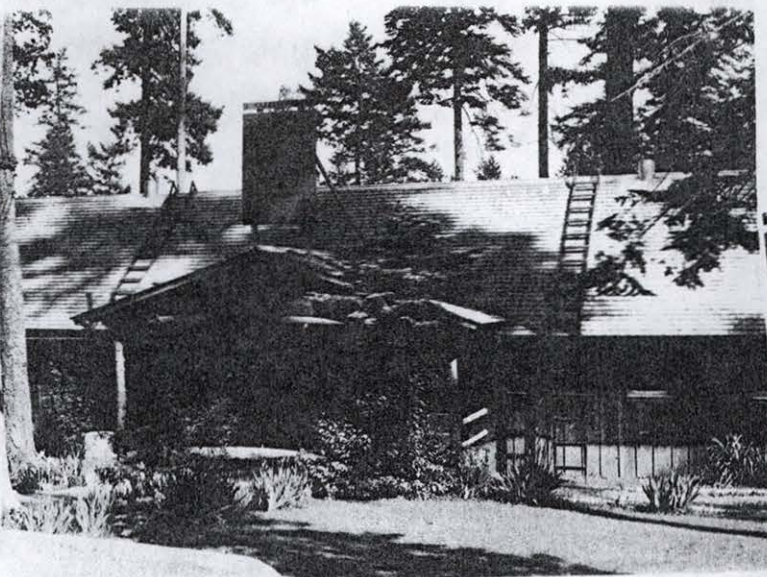
Safety First and Accident Board
