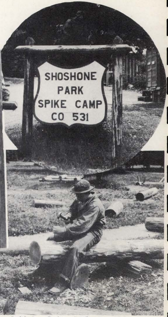
At Work on Parking Lot Barriers
