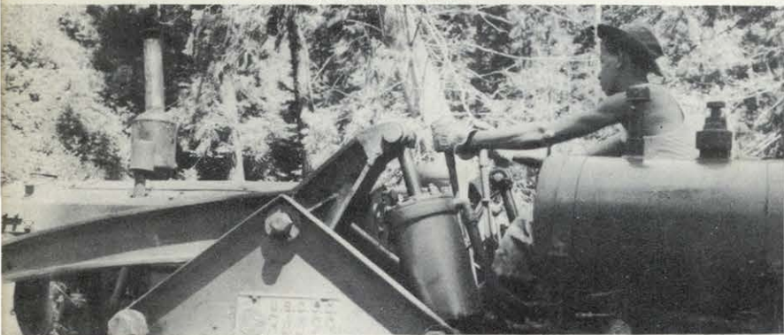
At Work on Big Creek Road
