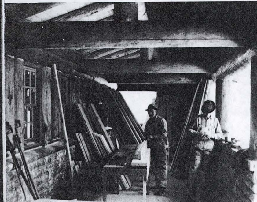
Construction Work on Rocky Point Community Lodge
