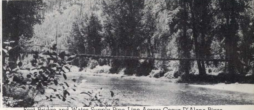
Foot Bridge and Water Supply Pipe Line Across Coeur D'Alene River
