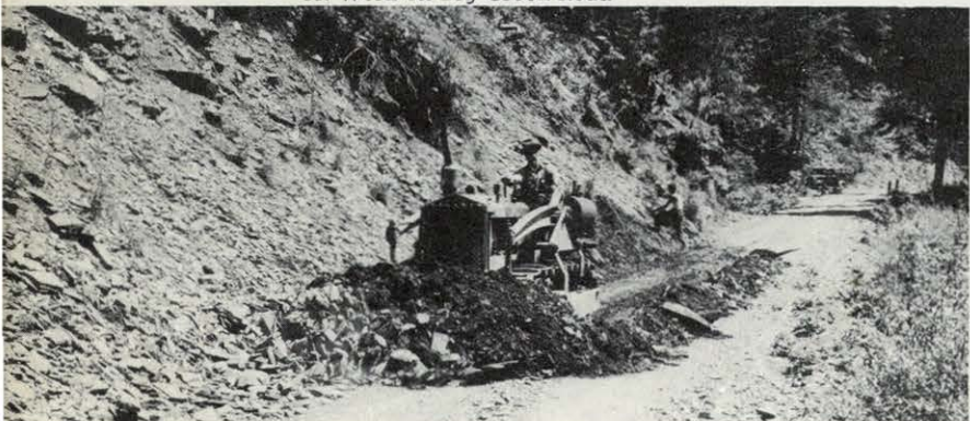
Maintenance of Big Creek Road
