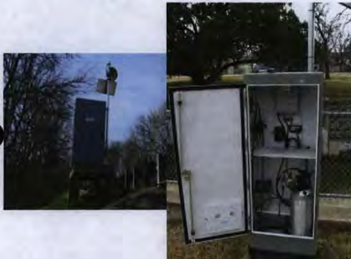
Figure 1. Examples of gage structures located at U.S. Geological Survey streamgaging stations.
