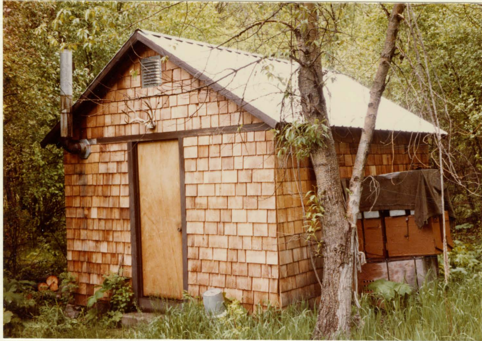
Photograph No. 3: View of subject bunkhouse.
