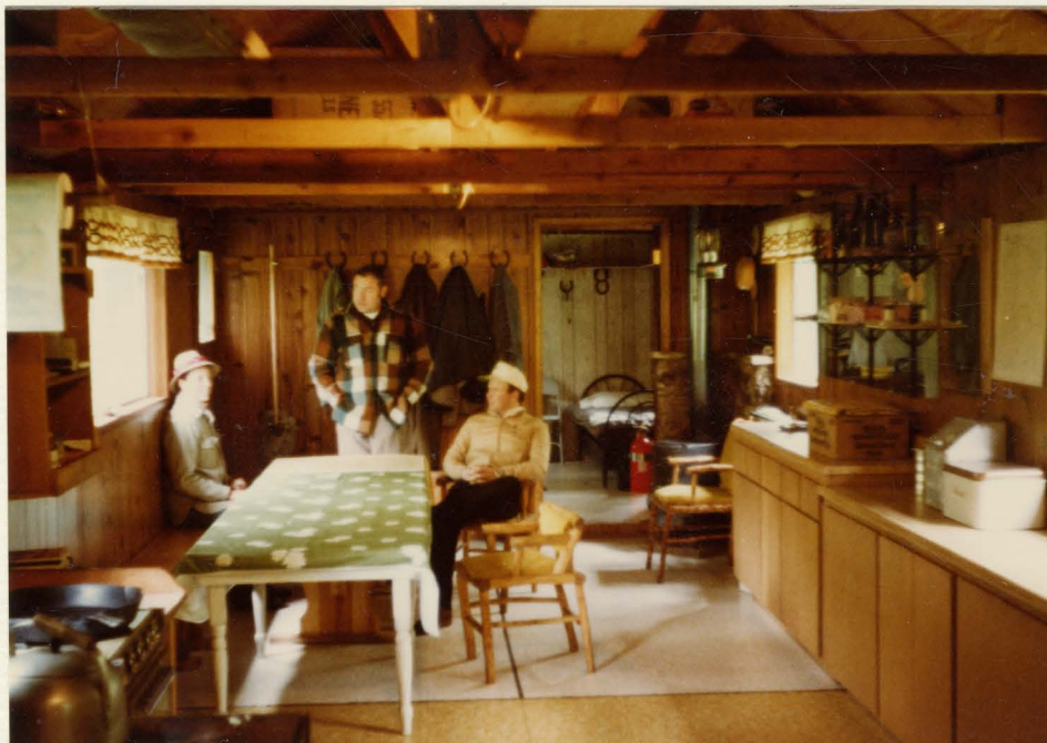
Photograph No. 2: Cookhouse interior looking west from main entrance.
