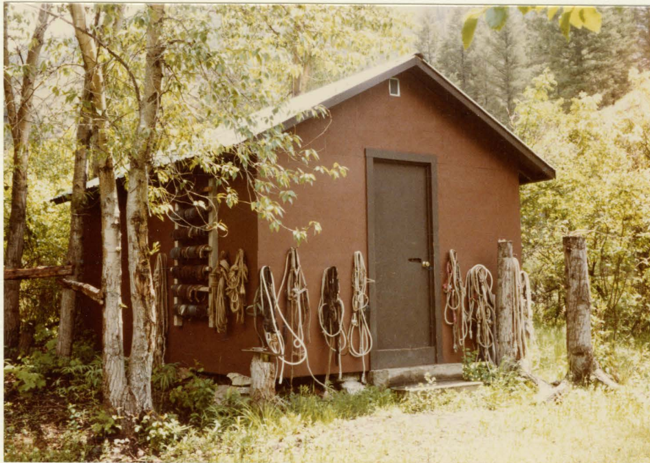
Photograph No. 4: View of subject tack room.
