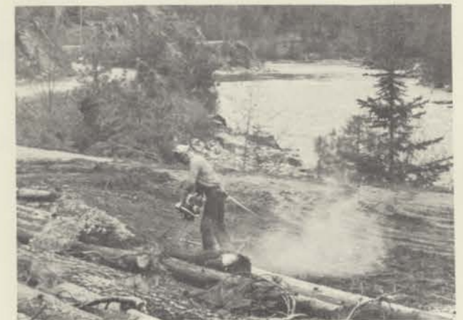
TIMBER CLEARING GETS UNDERWAY NEAR DAM SITE
