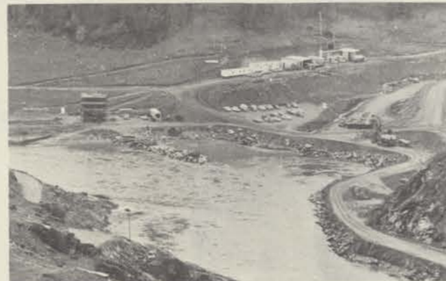
WORK AREA AT DWORSHAK TUNNEL
