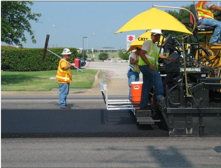
CORRECT SQUARE JOINT – END GATE DOWN
