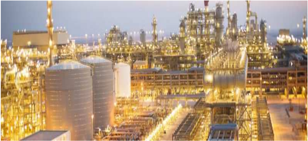
Figure 1.1. Shell's gas-to-liquids (GTL-FT) plant in Qatar. [www.shell.com].
