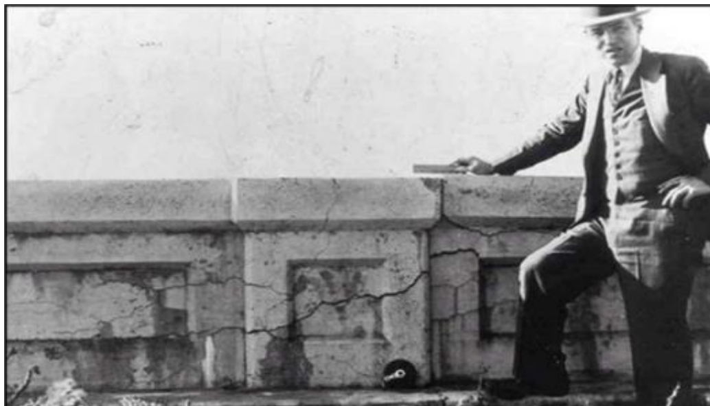
Figure 2.1 Typical Example of ASR in Concrete with Stanton
