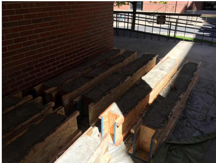
Figure 3.6: Beams after casting
