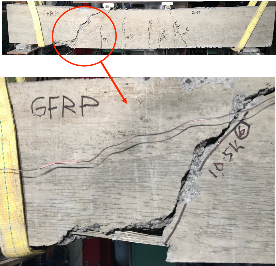
Figure 4.14: Failure mode of 10Cont-MN-2.5.
