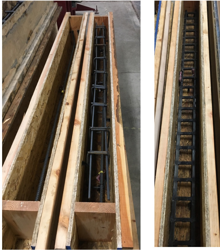
Figure 3.5: Beam 4 CONT-M8-2 formwork and reinforcement cage (left), and 8CF-M8-2.5 (right)
