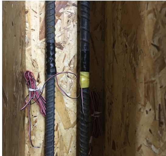
Figure 3.10: Strain gages installed at the bottom reinforcement.
