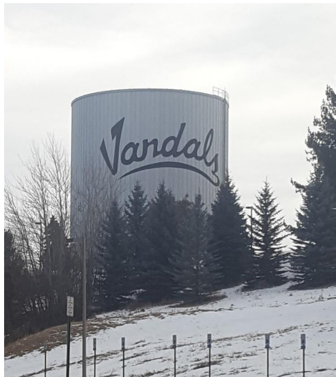
Figure 3.1: Cold TES tank located on the UI, Moscow campus, ID, USA
