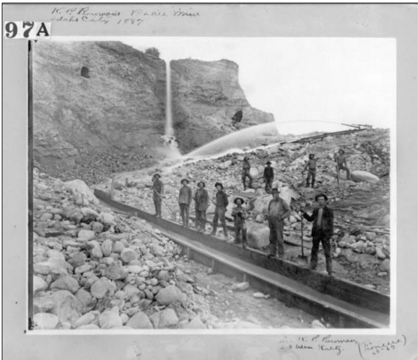
Figure 1.4. Hydraulic operations at the Plowman Mine in Idaho City. Two monitors can be seen on the far right. Their erosive power is evident in the volume of material stripped from East Hill behind them, which has become a receding scarp slope. The waterfall is a ground sluice delivering water from a ditch network to the wash pit below, which is then drained by the sluice box in the foreground. Idaho State Archives photo no. D 97-A.
