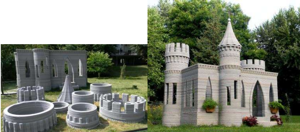
Figure 2-7: (Left) Printed pieces of castle [17]. (Right) Fully assembled castle [16].
