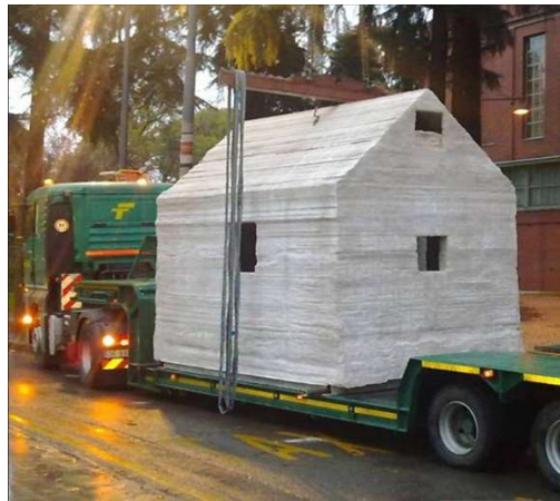
Figure 2-9:D-shape printed house [18].
