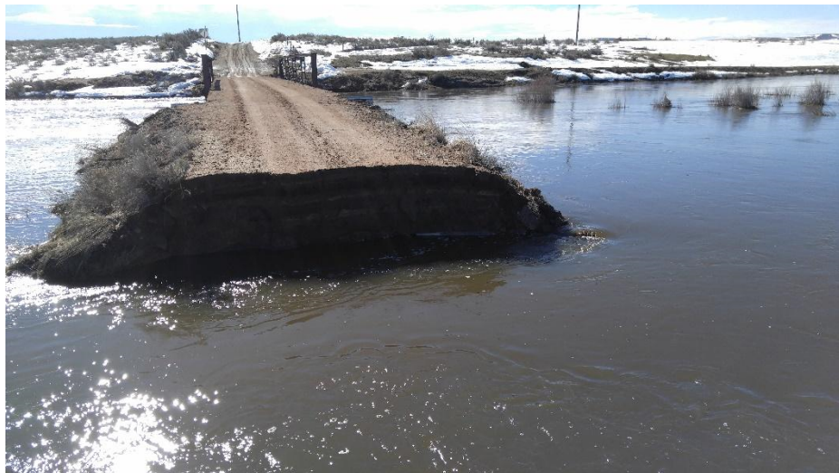
Figure 1.9. Camas Bridge in May 2017.
