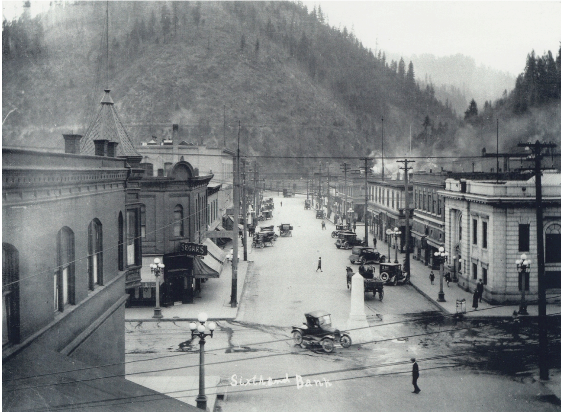
Figure 9: Looking north at the intersection of Sixth and Bank in Wallace in 1917. (Harry Graff Collection 637-19)
