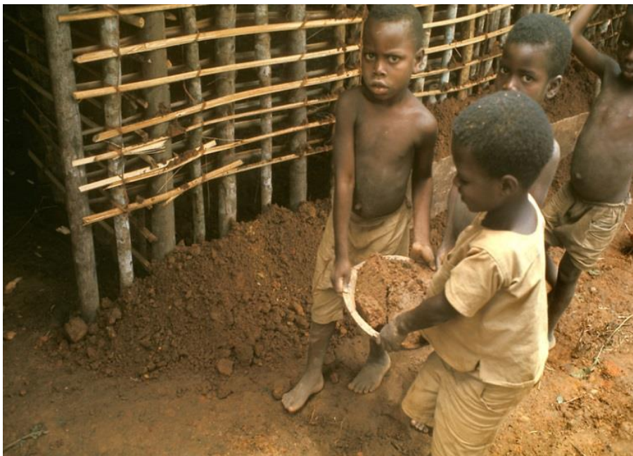
Figure 3: Children carrying mud, helping in the construction of a wattle-and-daub house.
