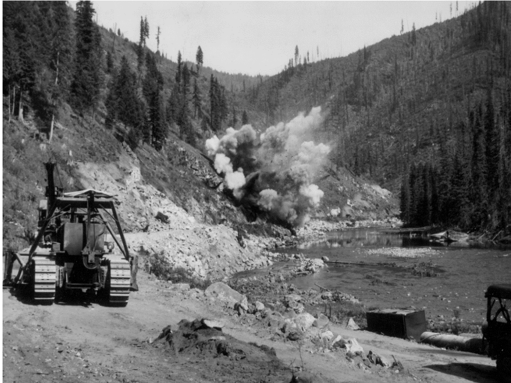
Figure 11. Highway 12 construction in the 1940's (U.S. Forest Service).
