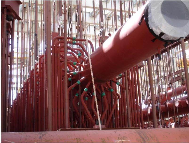
*Fig. 1.1.* Example of a boiler header pipe. [10]
