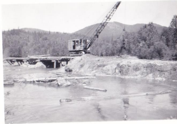
Figure 4.8. Date Unknown. Dragline crossing the bridge. 1945? (Emerald Creek Garnet, Ltd. 2017)
