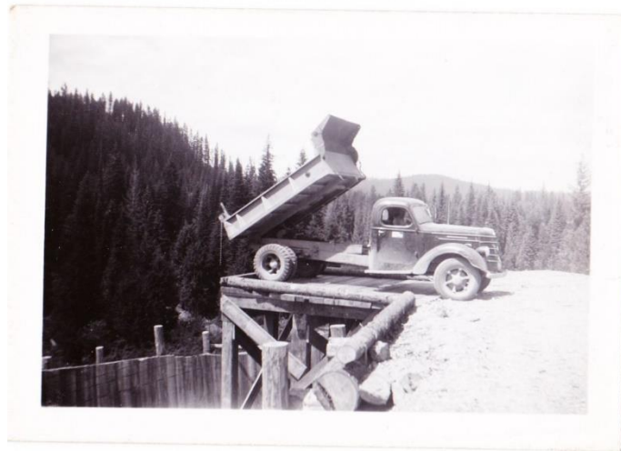
Figure 4.5. Date unknown, possibly 1940's. Dump truck unloading.
