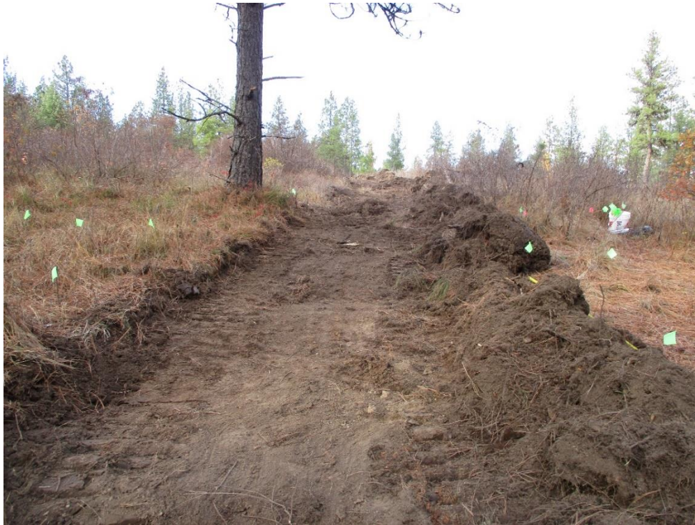
Figure 4.7: View of Unit 2, looking north, after the fireline was constructed
