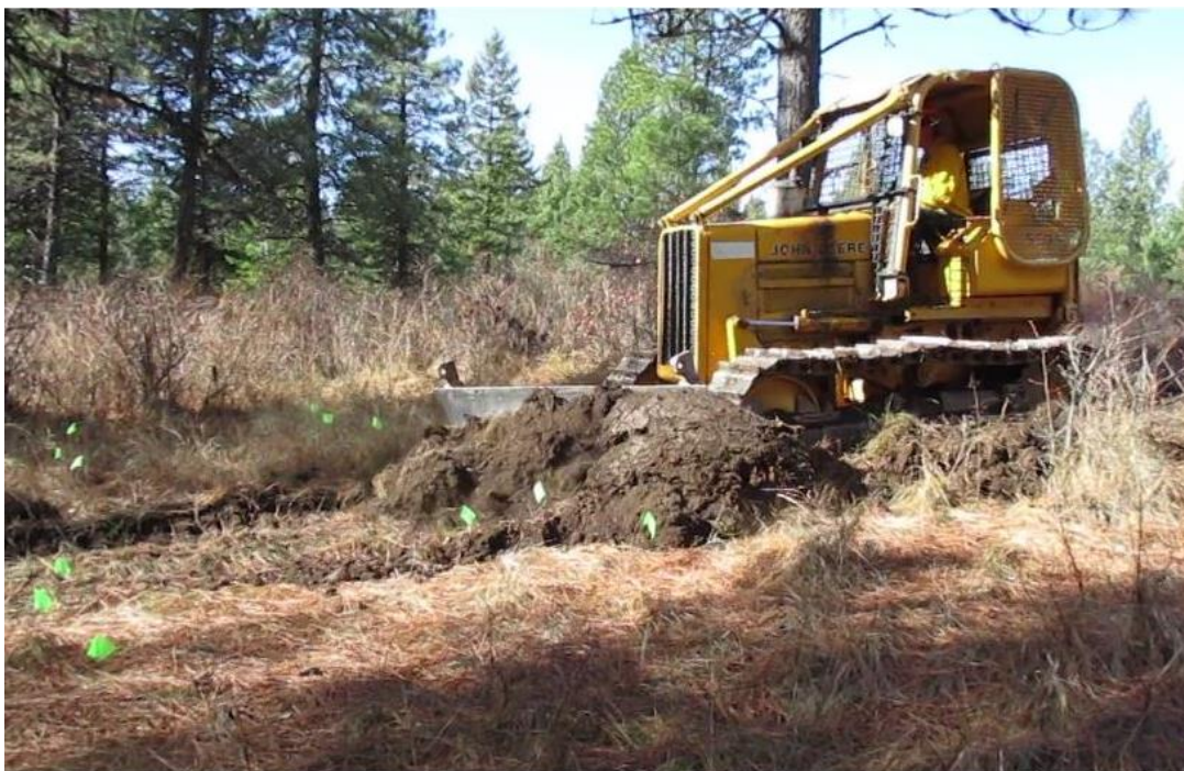
Figure 4.5: Construction of the fireline at Unit 2
